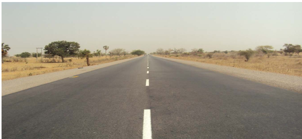
Picture 29: Completed Section of the Road
