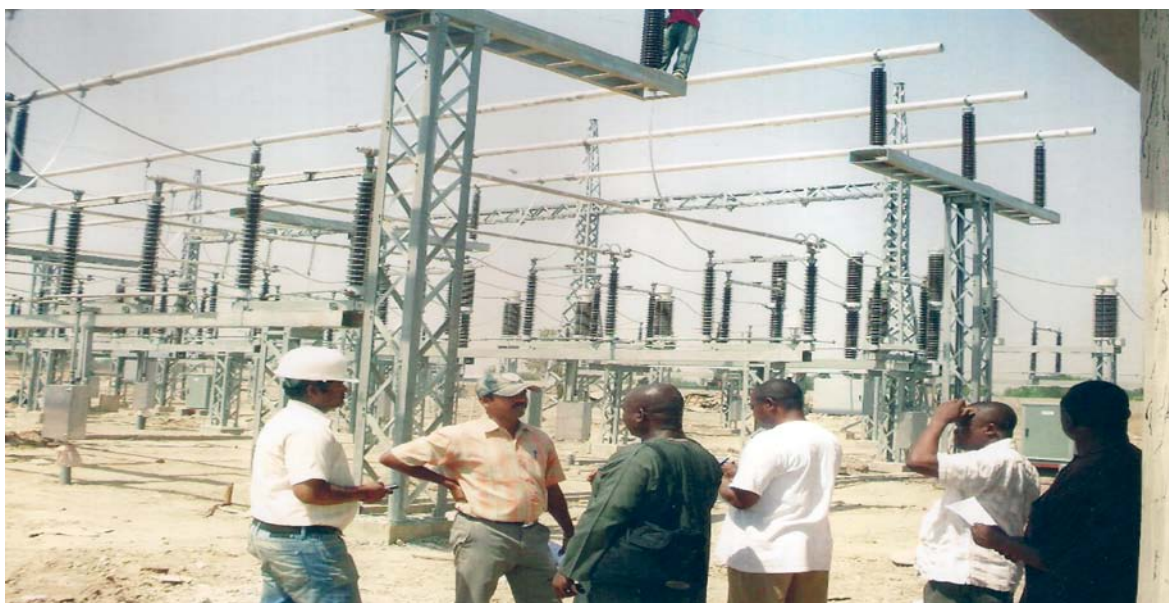
Picture 27: Ongoing Transmission Project at Yola Sub-Station
