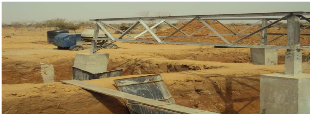
Picture 26: Construction Work at Katsina-Daura Power Project
