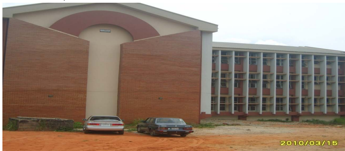
Picture 8: Completed Faculty Building for Engineering & Technology Wing B at Nnamdi Azikiwe University, Awka
