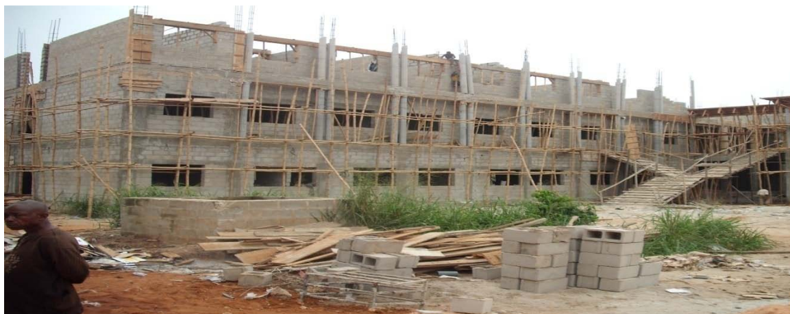
Picture 13: Ongoing Construction of Diagnostic Centre at Federal Medical Centre Owerri
