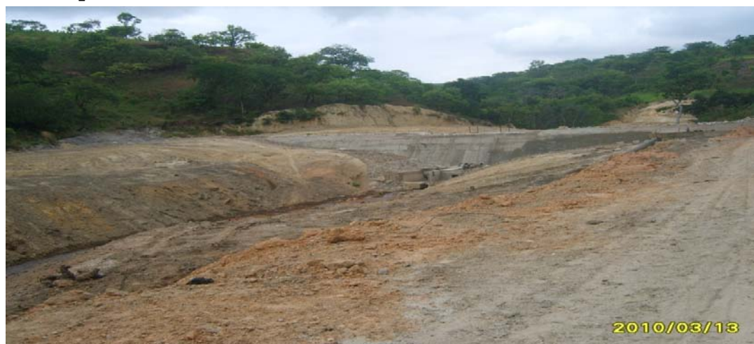
Picture 1: Ongoing Construction of Amechi-Awkunanaw Dam
