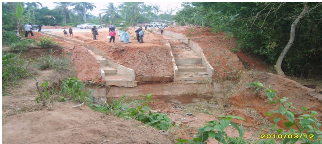
Picture 3: Ongoing Erosion Control Project in Ekenobizi, Imo State
