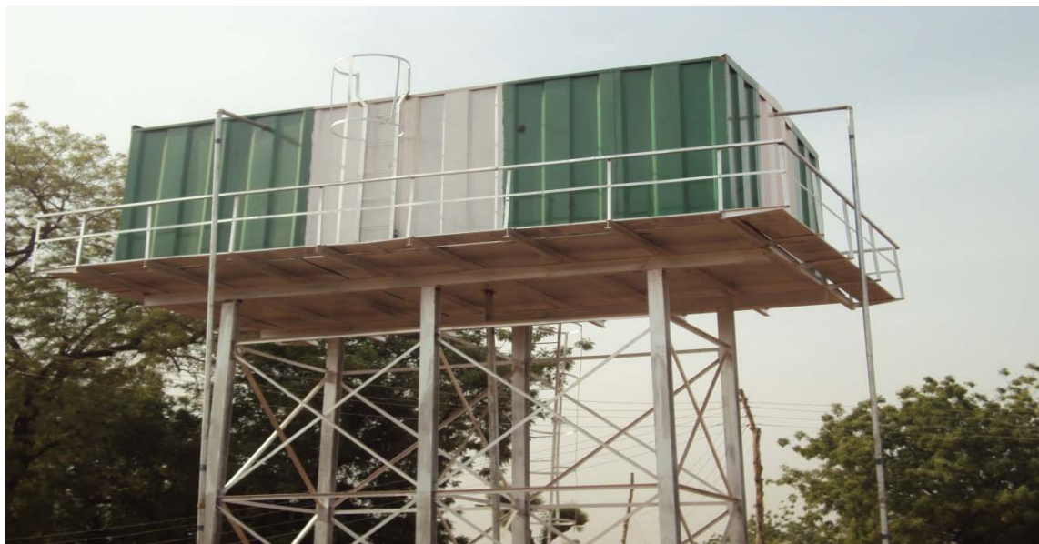
Picture 4 Completed Overhead Tank
