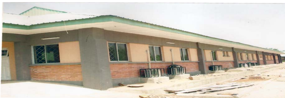
Picture 21: Completed CT Scan Block awaiting Installation of Machines
