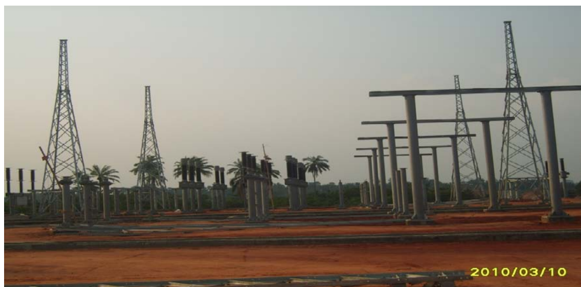
Picture 25: Ongoing Construction of 2x30/40MVA, 132/33KV Substation at Umuahia, Abia State
