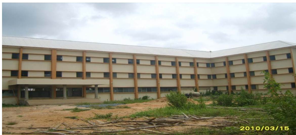
Picture 9: Newly Constructed Student Hostel at Nnamdi Azikiwe University, Awka, Anambra State
