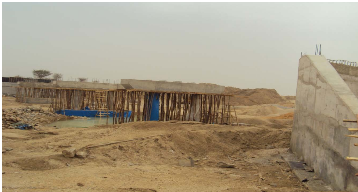
Picture7: Ongoing work on the Challawa Gorge Dam Spillway Crossing Bridge
