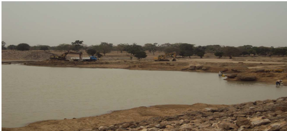
Picture 5: Ongoing work at the Dam
