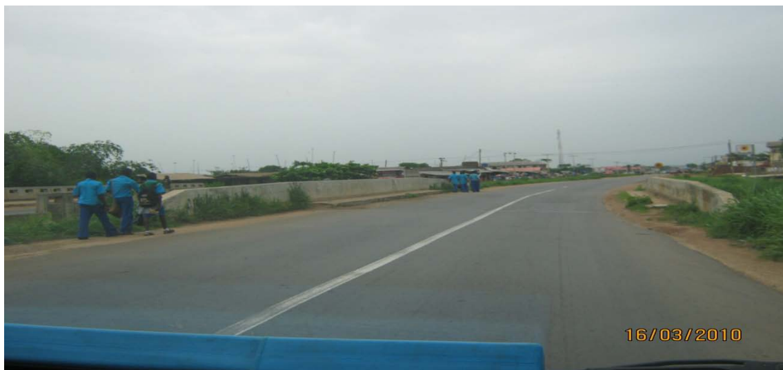
Picture 31: Construction work at Dualisation of Abeokuta-Otta Road
