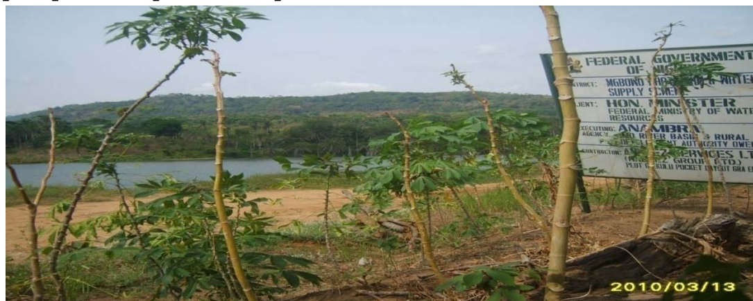
Picture 2: Constructed Dam Site at Mgbowo Water Scheme, Enugu
