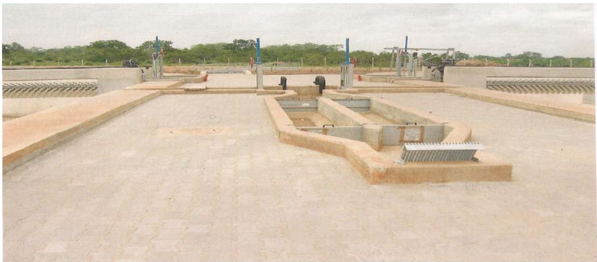
Picture 12: Sewage Treatment Plant at Ktampe District
