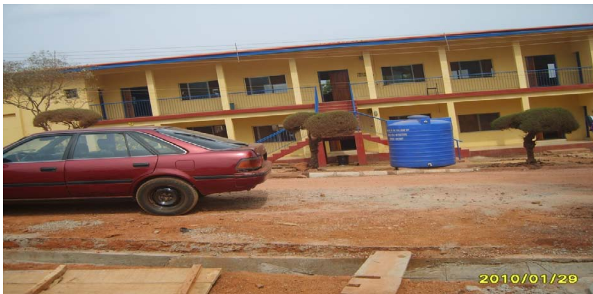
Picture 24: Rehabilitated Classroom Block at Police Intelligence School, Enugu
