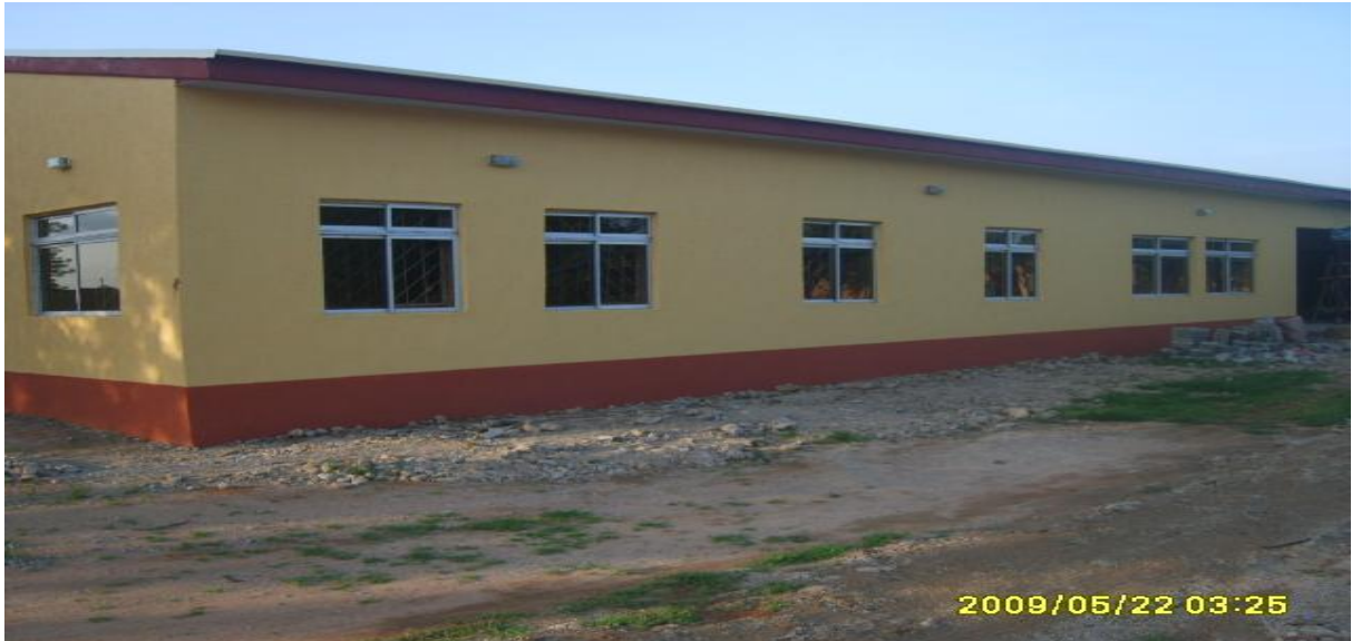
Picture 5: Completed Eye Unit section of the ENT complex at the Federal Medical Centre, Katsina
