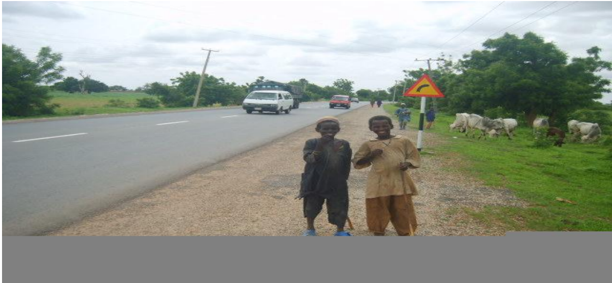
Picture 12: Rehabilitation of Talata Mafara–Sokoto Road Section III, Fully completed and in use
