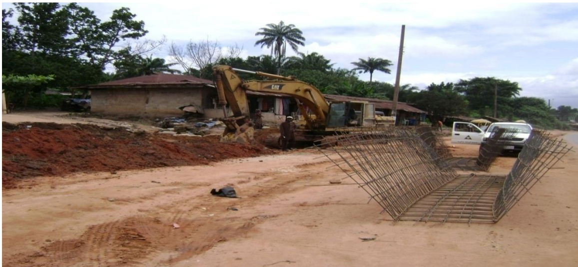
Picture 13: Ongoing Construction of Onitsha – Owerri Road Section I, Anambra/Imo States
