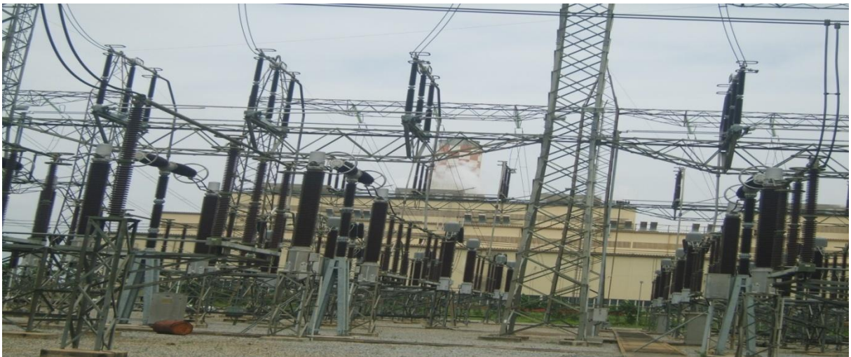
Picture 8: Completed Transmission – Egbin-Ikeja West/Benin Main 330KV D/C Line and S/S
