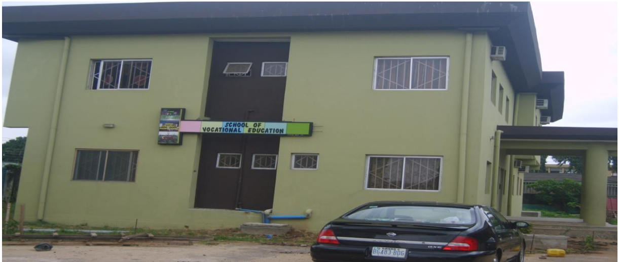
Picture 2: Completed Office Building for School of Vocational Education (SVE) in College of Education (Technical) Akoka, Lagos
