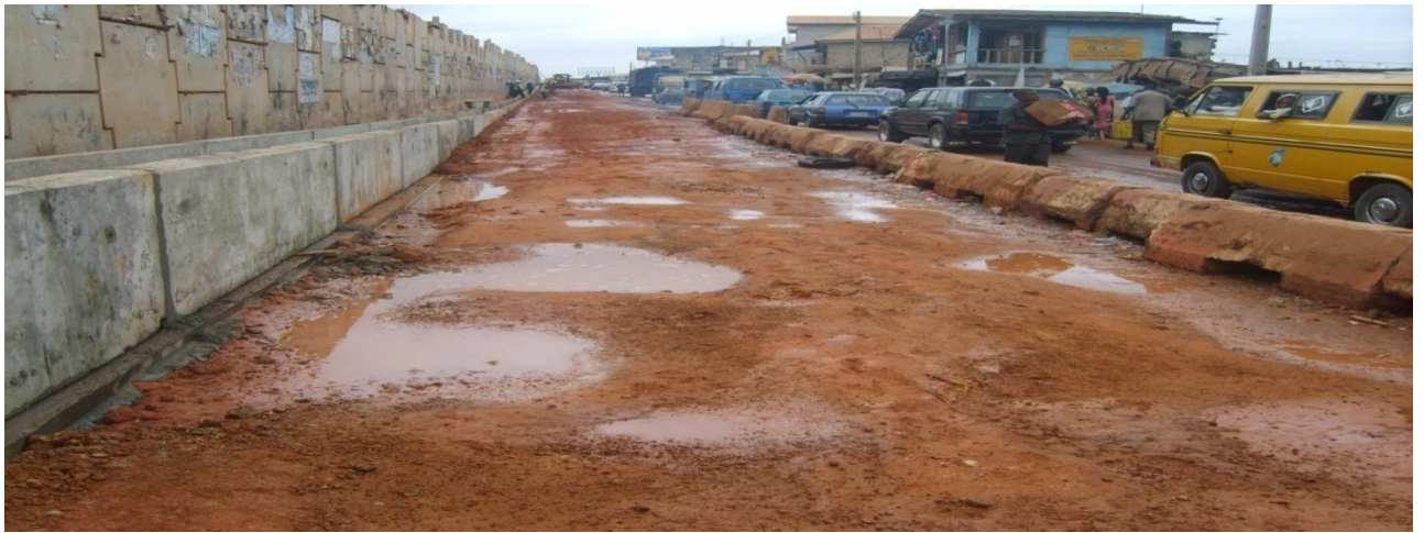
Picture 10: On-going Construction of Fly-over Bridge at Otta-Abeokuta Road, Ogun State
