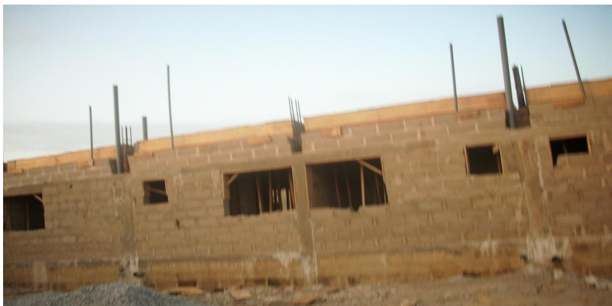
Picture 18: Ongoing Construction of Main Administrative Block, NSCDC Academy, Abuja.
