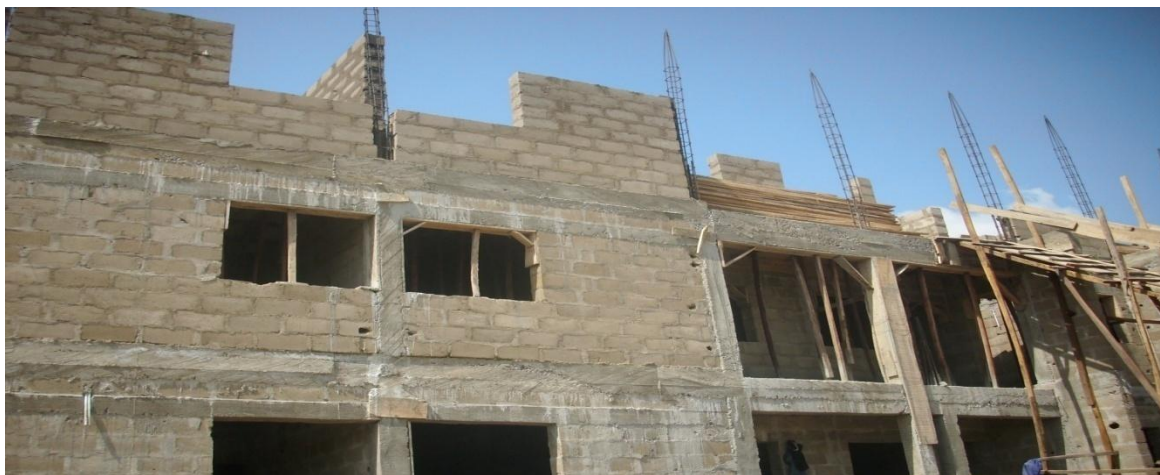
Picture 12: Staff Quarters under Construction National Fire Service Academy, Sheda, Abuja
