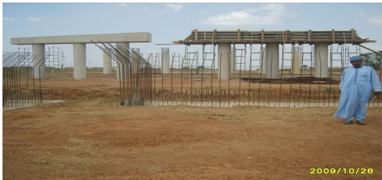
Picture 21: Ongoing Construction of Bridges at Kano Western Bypass Road Project
