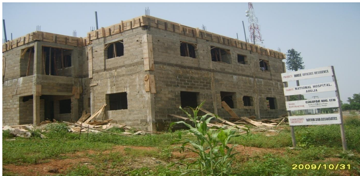
Picture 19: Ongoing Construction of House Officers Quarters at National Hospital, Abuja
