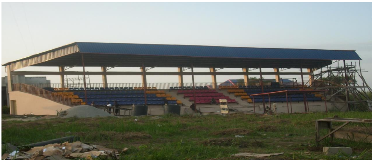
Picture 15: Ongoing Construction of Parade Ground, NSCDC Academy, Abuja.
