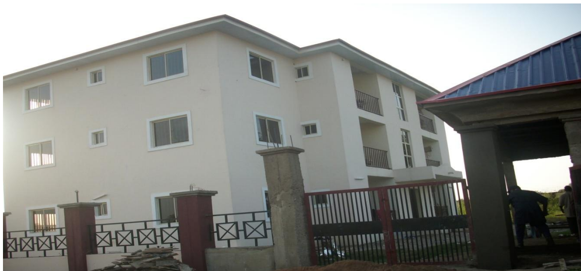
Picture 13: Completed 6-Unit of 2 Bedroom Flat of 2 Storey, NSCDC Academy, Abuja.
