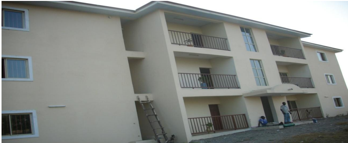
Picture 14: Completed 6-Unit of 3 Bedrooms Flat of 2 Storeys, NSCDC Academy, Abuja.
