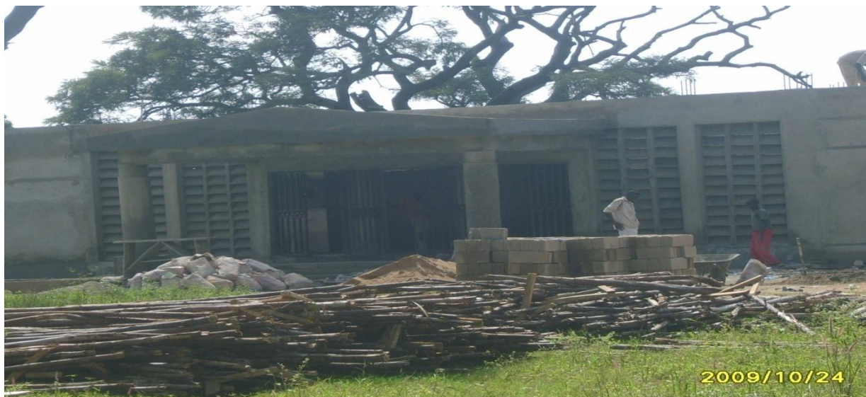
Picture 4: Ongoing Construction of Classroom at Federal Polytechnic, Kaduna (Permanent Site)
