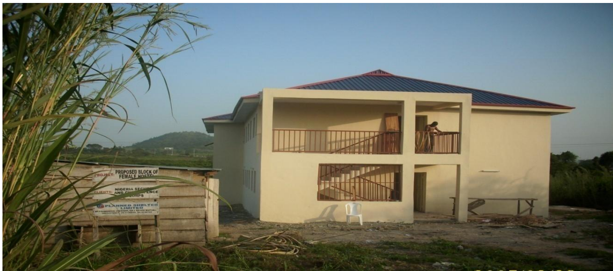
Picture 17: Completed Male Hostel Block, NSCDC Academy, Abuja
