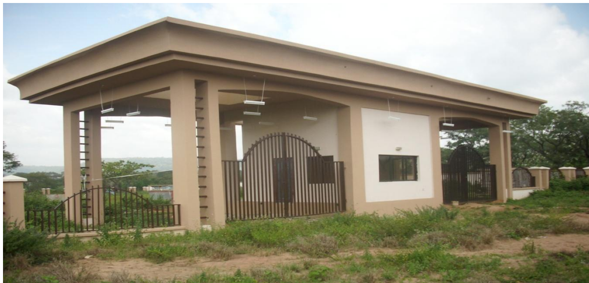
Picture 20: Completed Fencing and Gate House, NBTI Headquarters, Abuja
