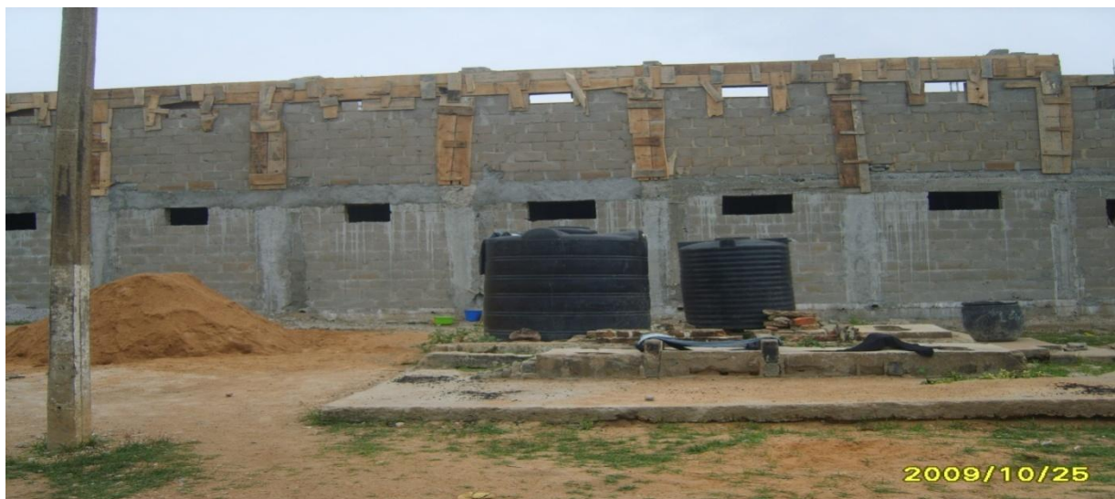
Picture 9: Ongoing Construction of Storey Cell Block for CCC in Kaduna
