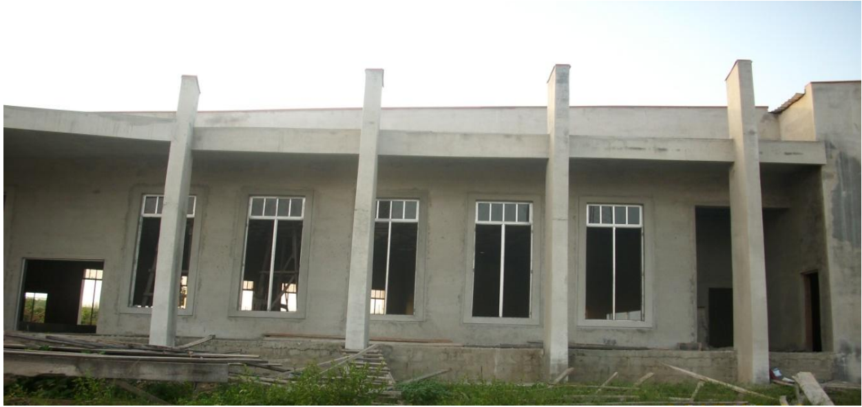
Picture 16: Ongoing Construction of Auditorium, NSCDC Academy, Abuja.
