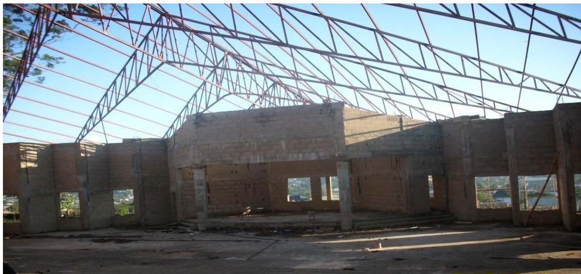
Picture 8: Ongoing Construction of Auditorium, National Orthopaedic Hospital, Enugu.
