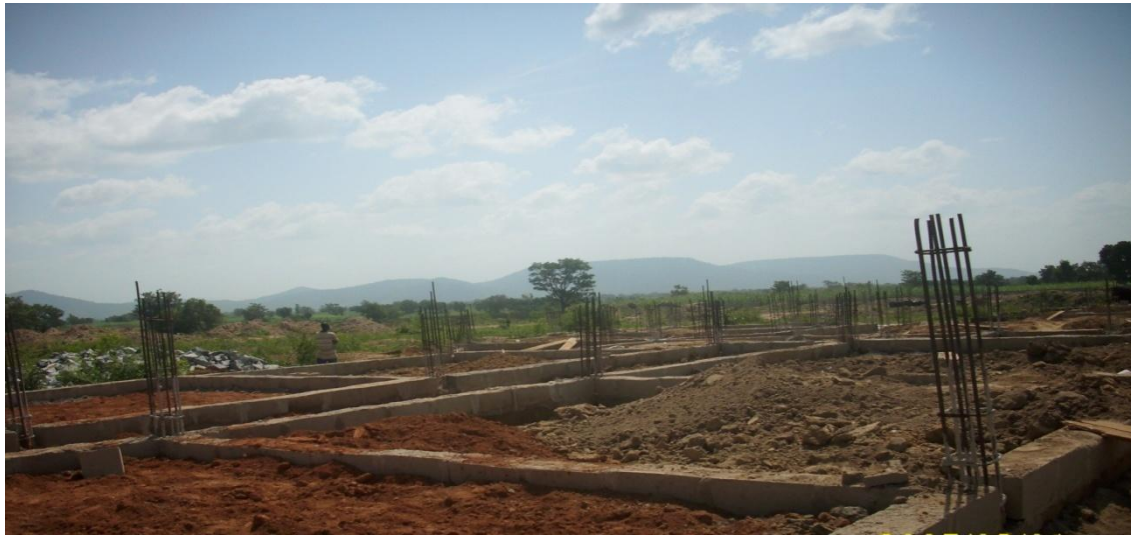
Picture 11: Administrative Block foundation being filled
