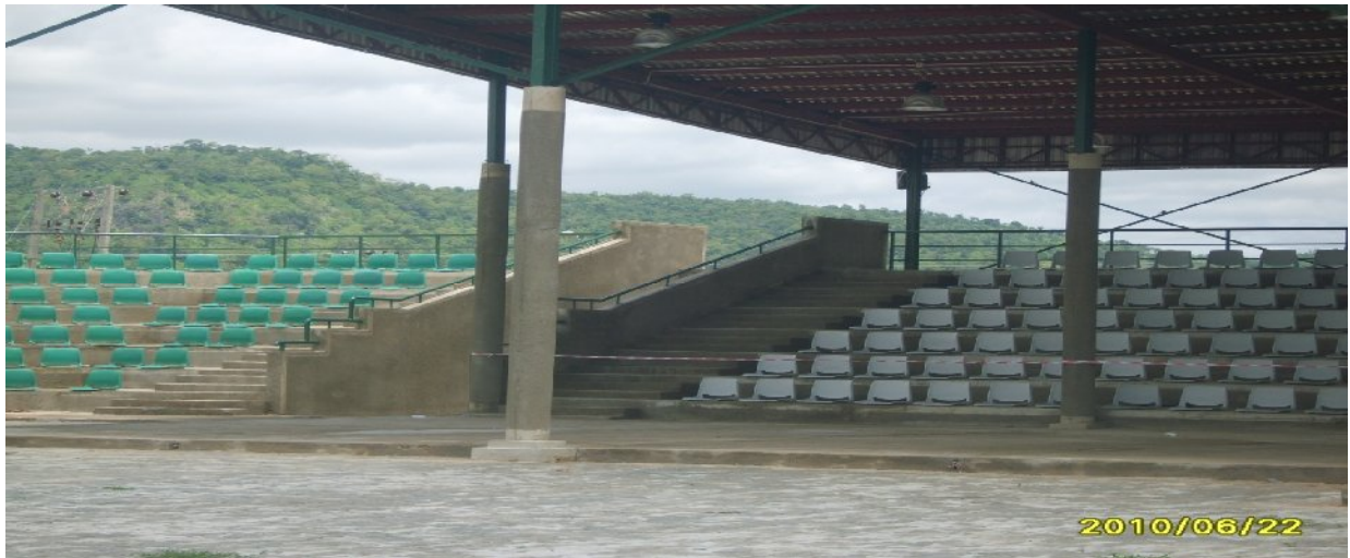
Picture 9: On-going construction of Convocation Square at the University of Abuja
