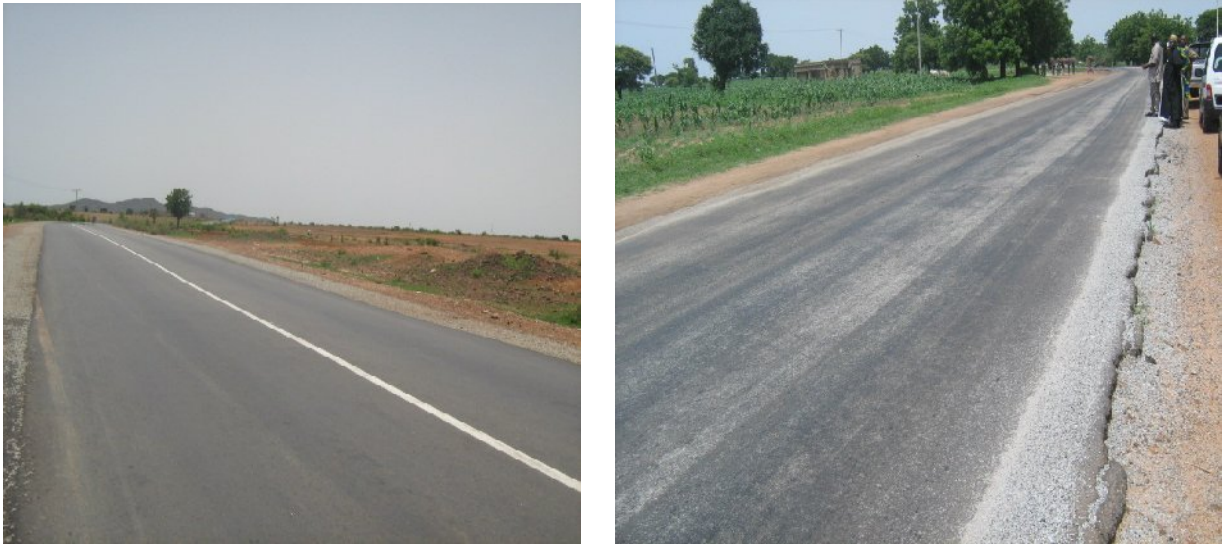
Picture 17 & 18: Rehabilitation of Funtua-Gusau-Sokoto Road
