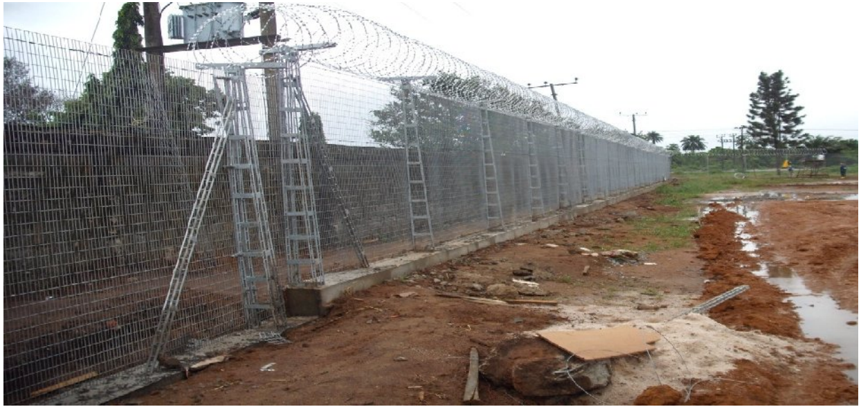
Picture 28: Bi-lattice metal fence at the Port-Harcourt International Airport
