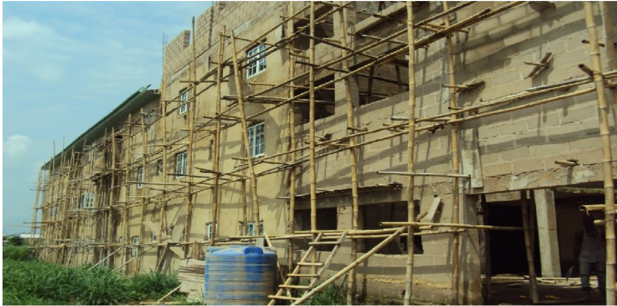
Picture 1: Ongoing work at the multipurpose ward
