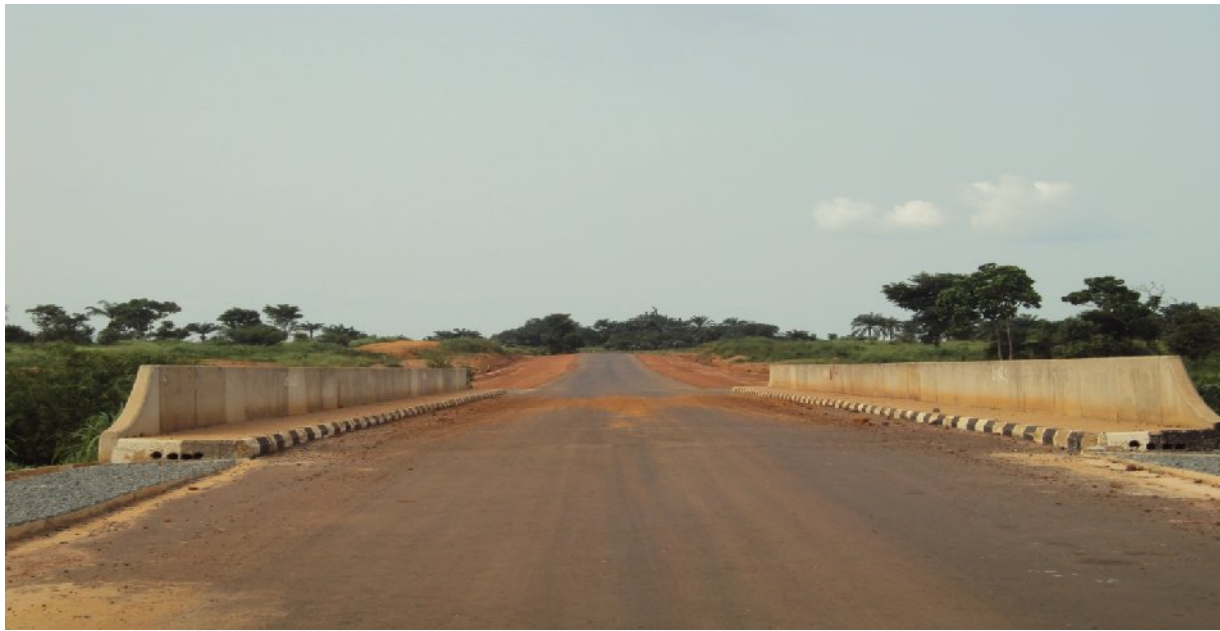
Picture 16: One of the completed bridges on the Obiozara-Enugu Road
