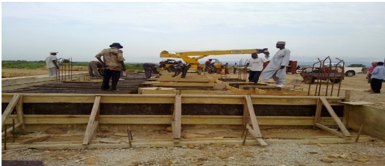
Picture 4: Ongoing work at Kaltungo earth dam
