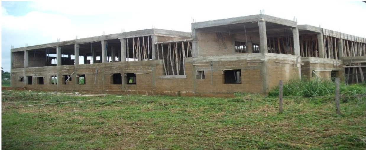
Picture 3: Three storey medical ward building at UUTH
