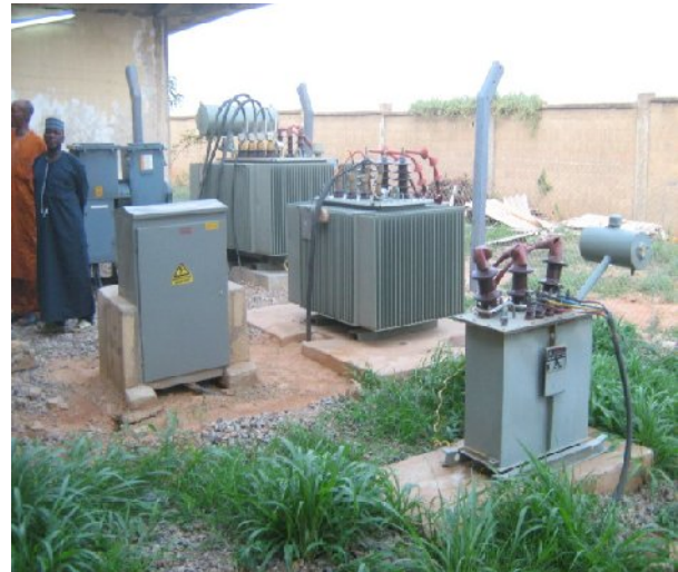
Picture 27 (a & b): Power upgrading works at the Kano International Airport
