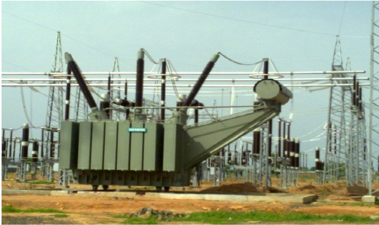
Picture 21: Ongoing work at the Jalingo Transmission Line
