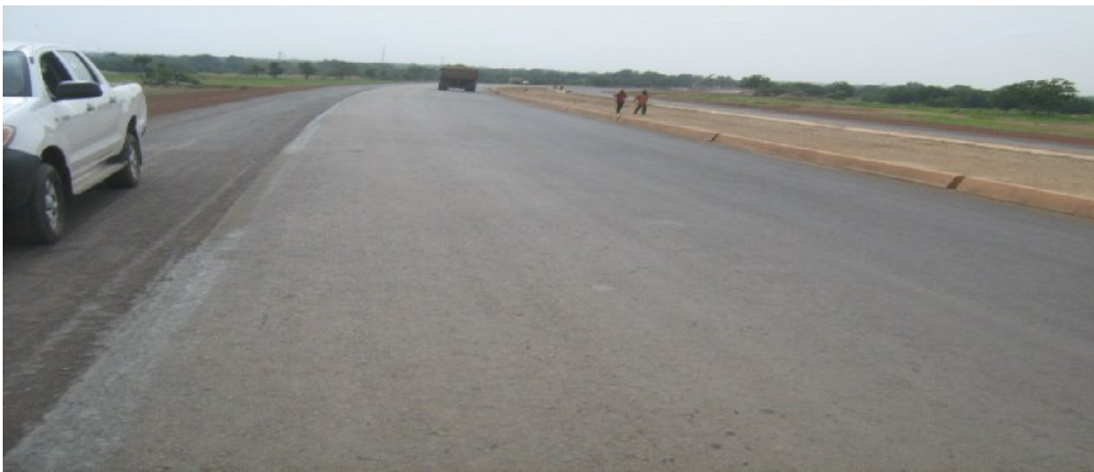
Picture 19b: Work on the ongoing Kano western Bye-pass
