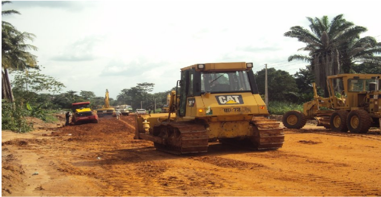
Picture 15: Ongoing work on the Obiozara-Enugu Road
