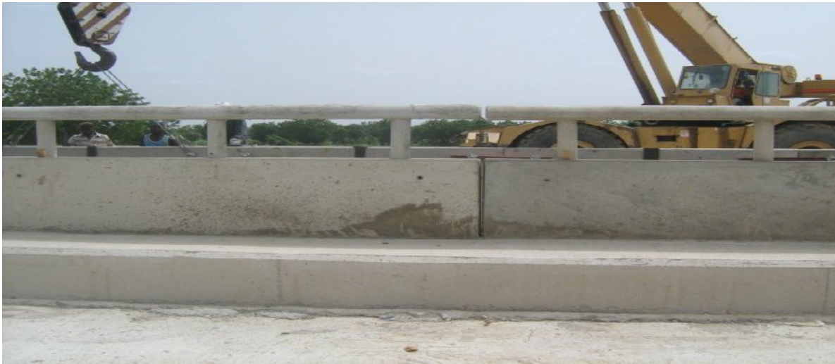
Picture 19a: Work on the ongoing Kano Western Bye-pass
