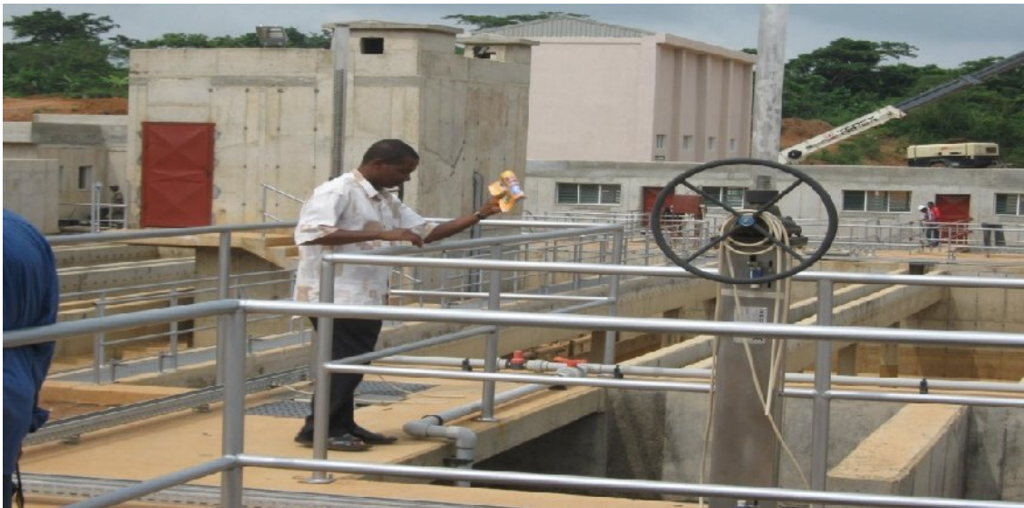
Picture 6: Ongoing water treatment plant at Owena Dam
