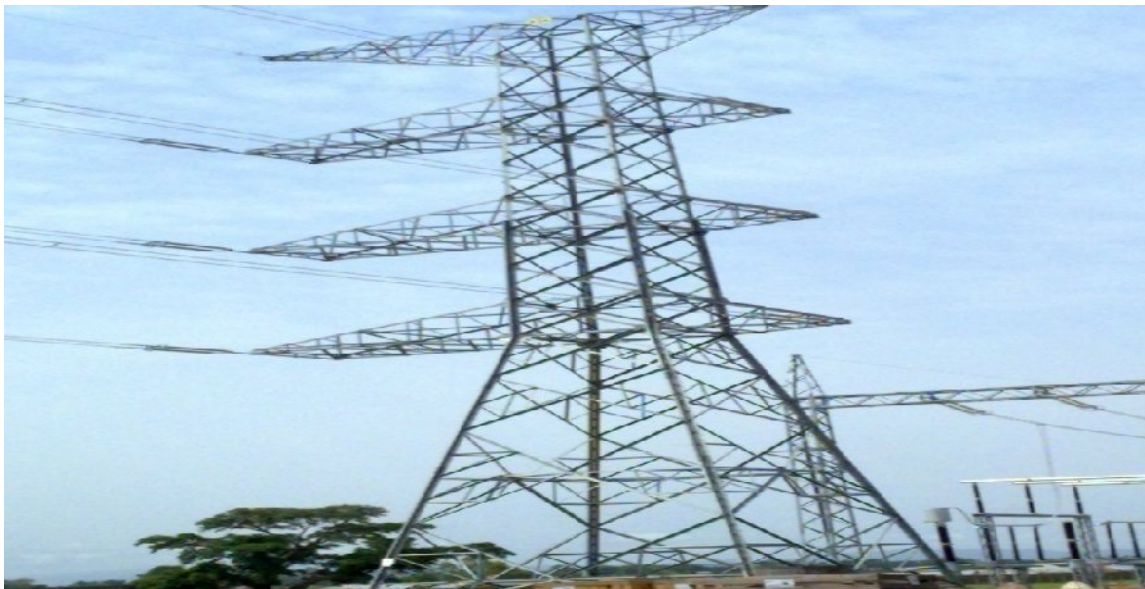
Picture 22: On-Going Work at Damaturu Transmission Line
