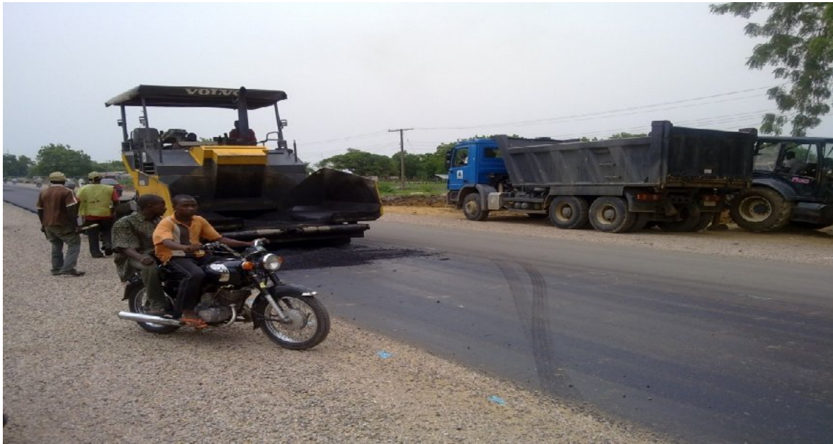
Picture 10: On-going work on Numan -Yola road
