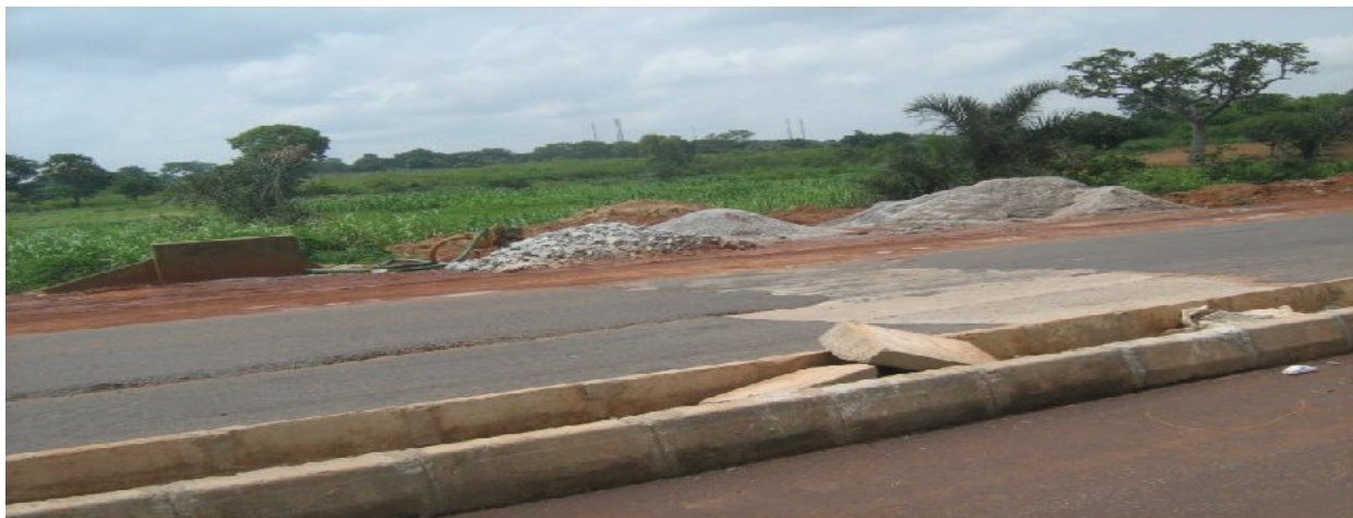
Picture 20 (a & b): Rehabilitation of access road to the Kaduna refinery
