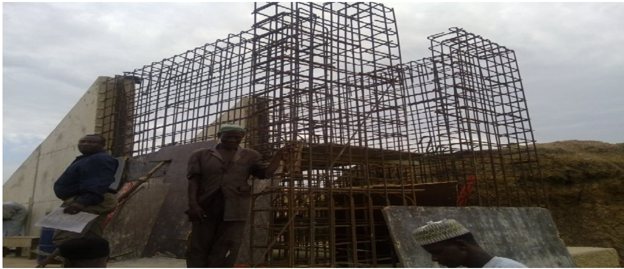
Picture 11: Construction of bridge at the Gombe Bye-pass
