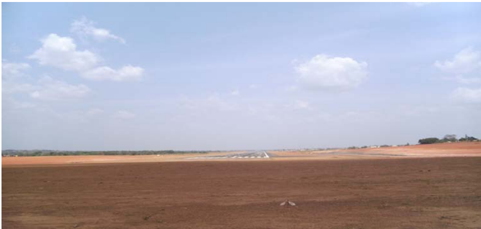
Picture 19: On-going expansion and resurfacing of Enugu Airport runway
