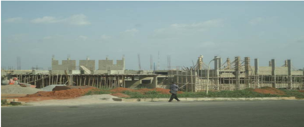
Picture 29: On – going construction of 2,500 Seat Auditorium
