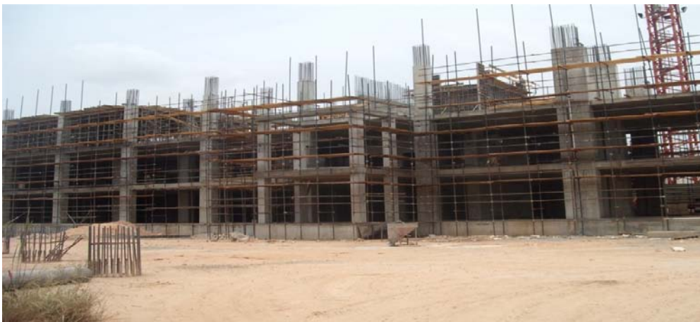
Picture 5: Ongoing construction at Nigerian Cultural Center and Millennium Towers, Abuja.
