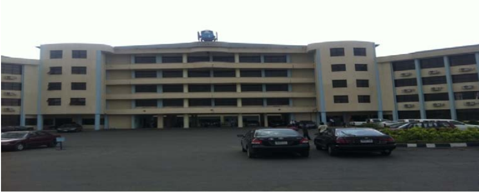
Picture 24: Completed Central Administrative/Senate Building at the University of Portharcourt
