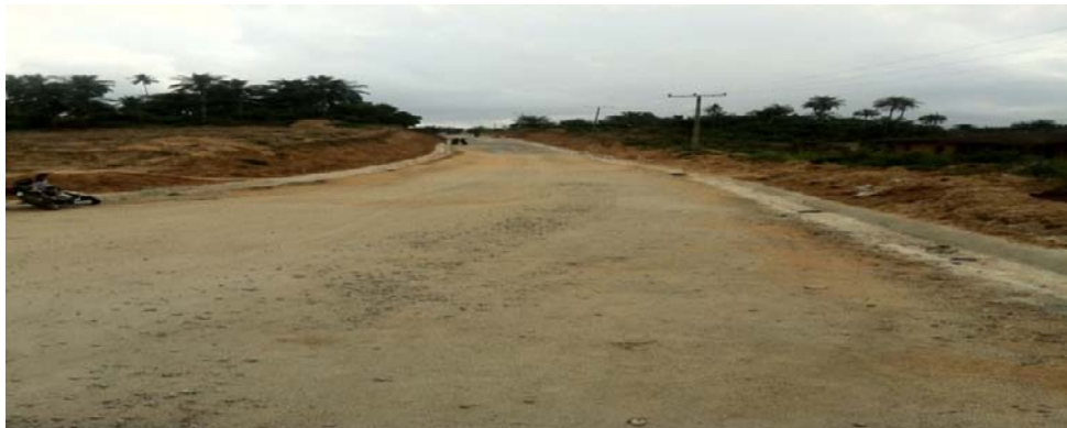
Picture 21: Ongoing construction of Main Access Road at NIFOR Institute, Benin
