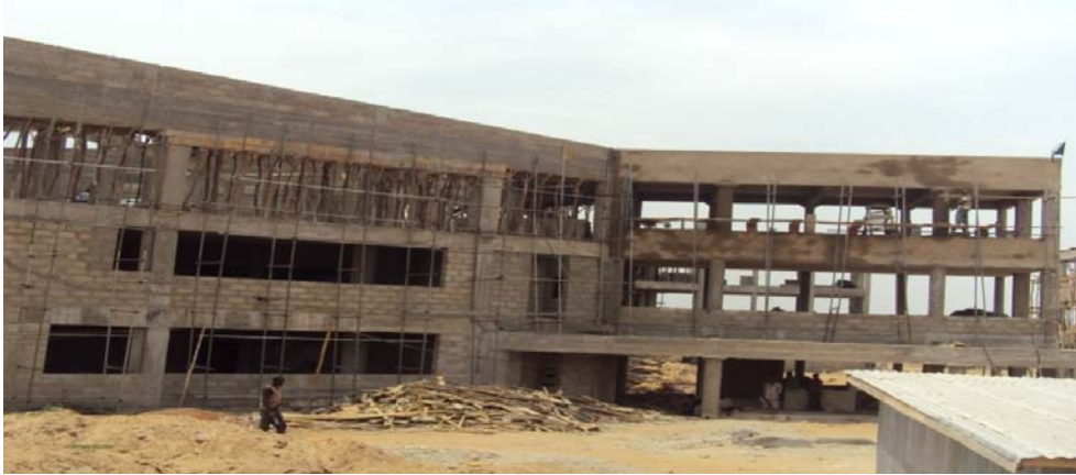
Picture 25: On-Going Work at ICT Centre, Federal University of Technology, Minna
