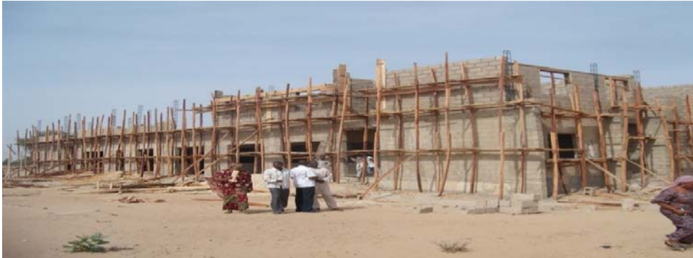
Picture 33: Ongoing Administrative Block Building at Federal Medical centre Nguru
