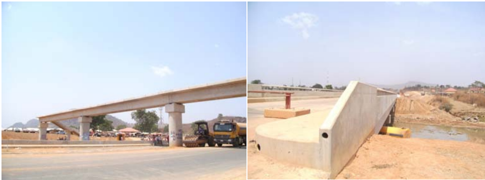
Picture 3a: Pedestrian Bridge at the rehabilitated and expanded Kubwa Expressway
