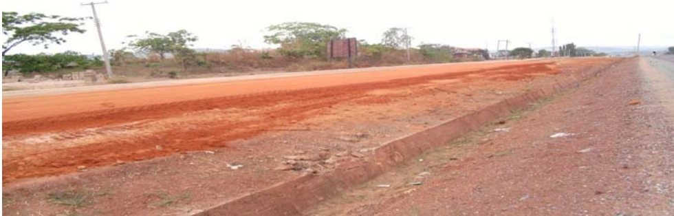
Picture 9: Rehabilitation of 9 th Mile Enugu-Port Harcourt Dual Carriageway in Enugu
