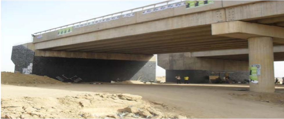
Picture 13: completed fly over bridge of the Kano Western Bye Pass
