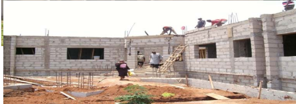
Picture 28: Construction of 20 room Guest house at FUTO, Owerri
