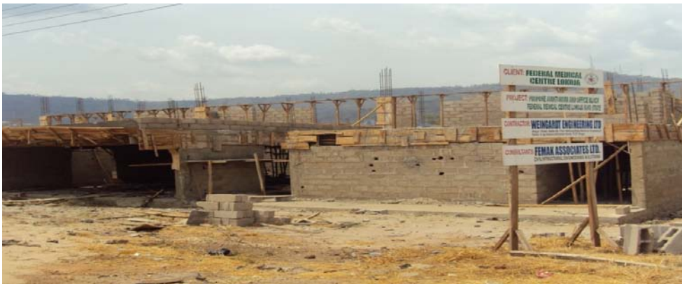
Picture 32: Ongoing Construction of Auditorium Complex
