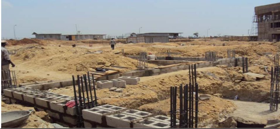
Picture 26: Foundation work at the Department of Computer Engineering.
