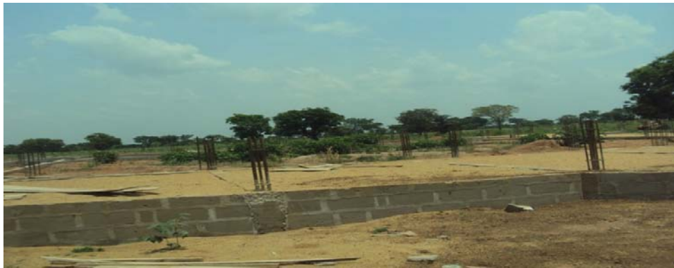
Picture 31: Ongoing Foundation for Construction of GOPD
