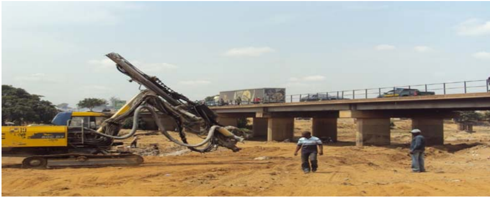
Picture 6: On-going construction work at Gwagwalada Bridge..
