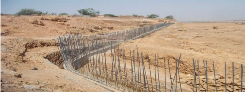
Picture 23: Nafada Erosion Control Project in Nafada LGA, Gombe State.
