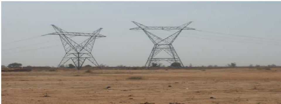
Picture 17: Transmission Project Gombe-Damaturu-Maiduguri 330KV TRX line
