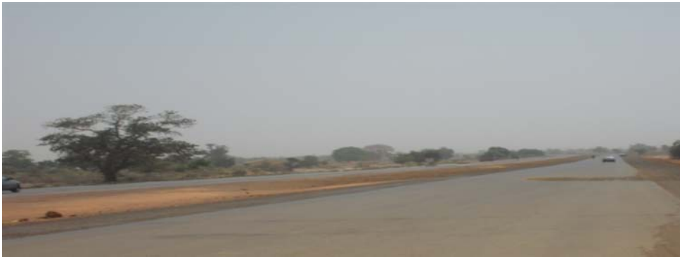
Picture 10: Ongoing work on dualisation of Kano-Maiduguri road, Section III (Azare-Potiskum).
