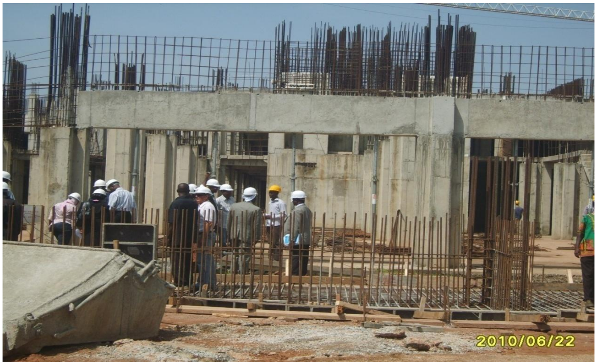
Picture 12: On-going Construction of National Library Building Headquarters, Abuja
