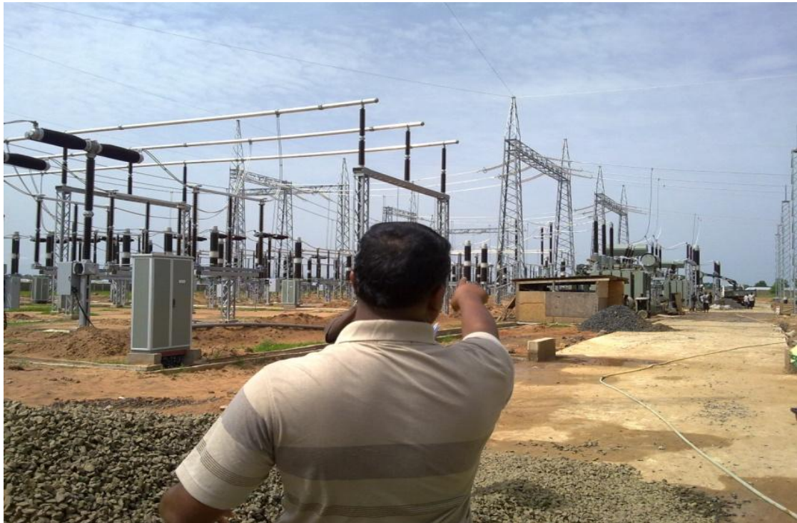
Picture 16: Ongoing work at Yola Sub-Station
