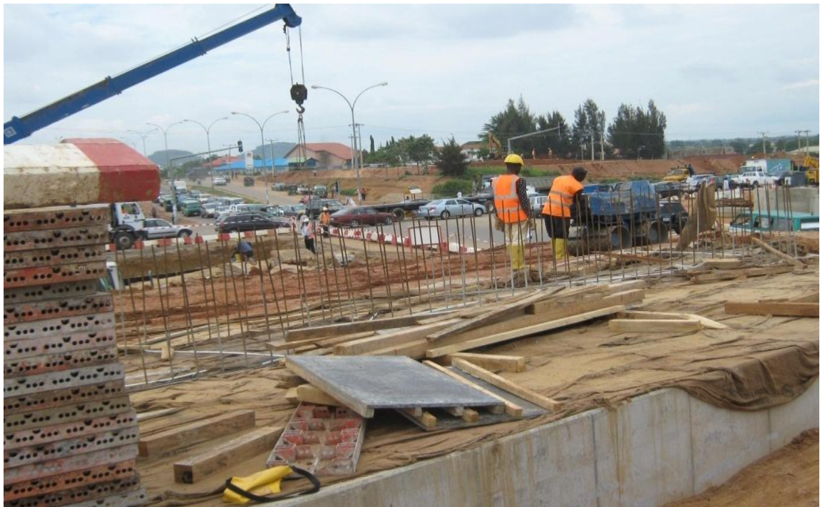
Picture 8: Ongoing Construction of Ring Road II / Arterial N5 Interchange
