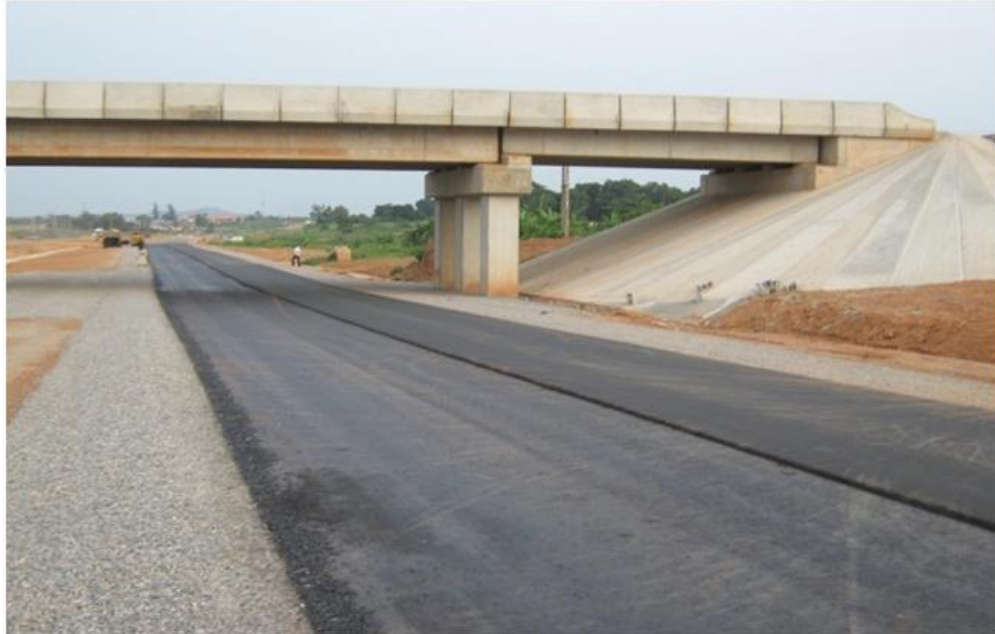
Picture 1: Ongoing construction of 2 nd flyover bridge over the Ibadan-Ilorin Road
