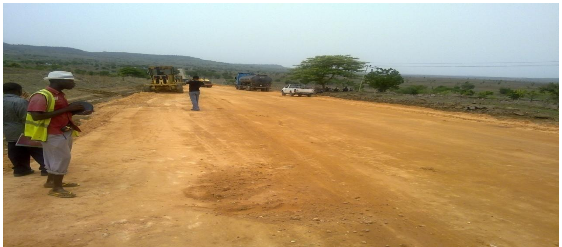
Picture 3: Ongoing work on Rehabilitation of Gombe-Numan-Yola Road, Section 2
