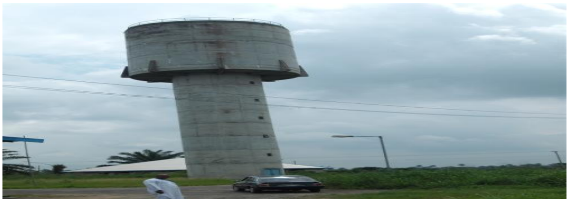
Picture 6: Akwa-Ibom water project
