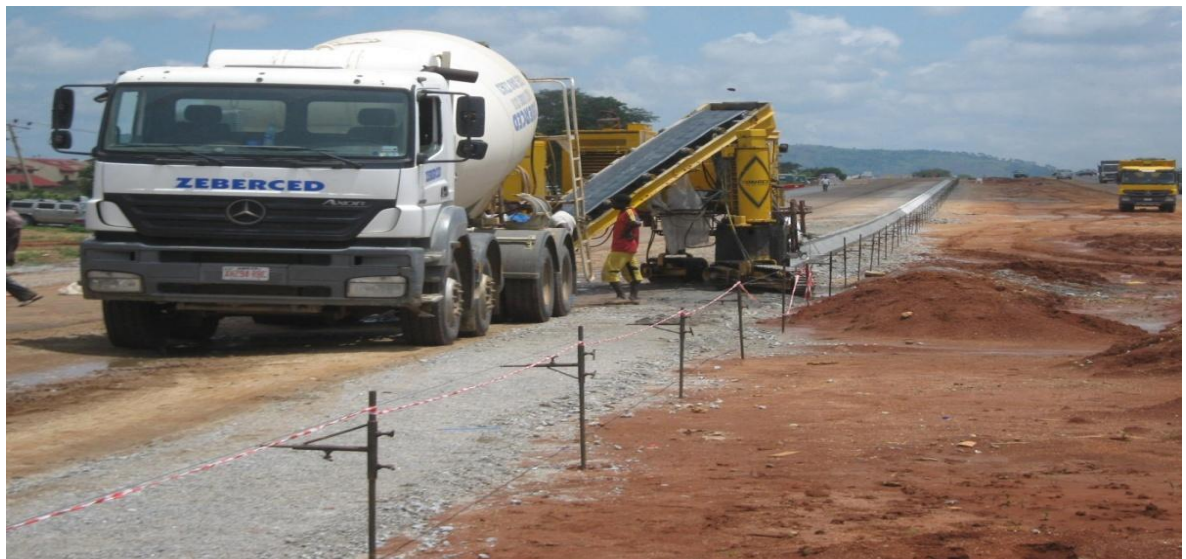
Picture 9: Kerb Stones Work in Progress at Lot II Service Carriageway
