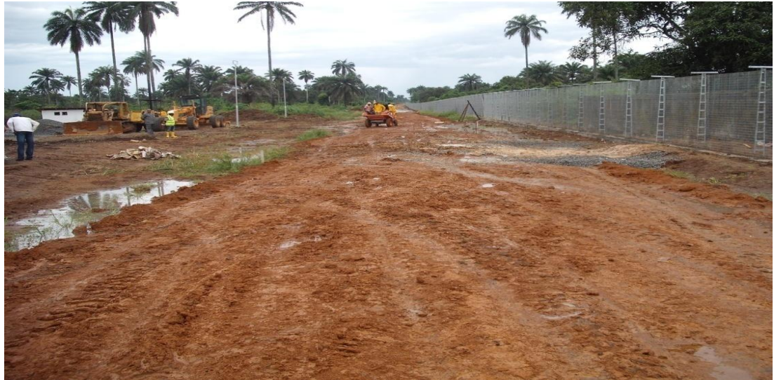
Picture 7: On – going construction of Asphalt Road at Port-Harcourt International Airport
