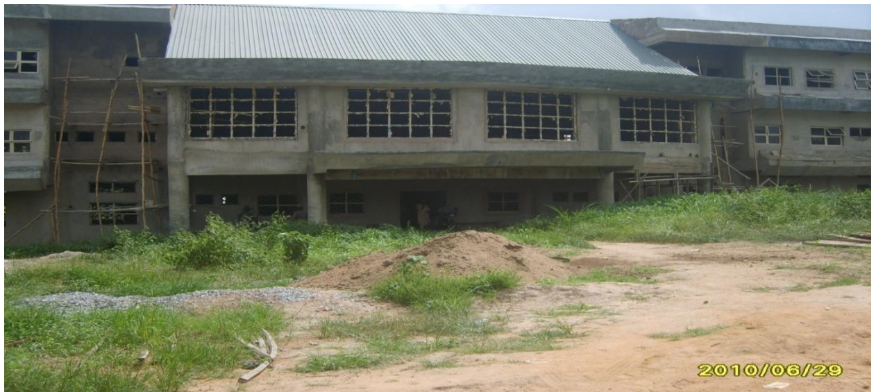
Picture 14: On-going Construction of FBSS at the University of Ilorin
