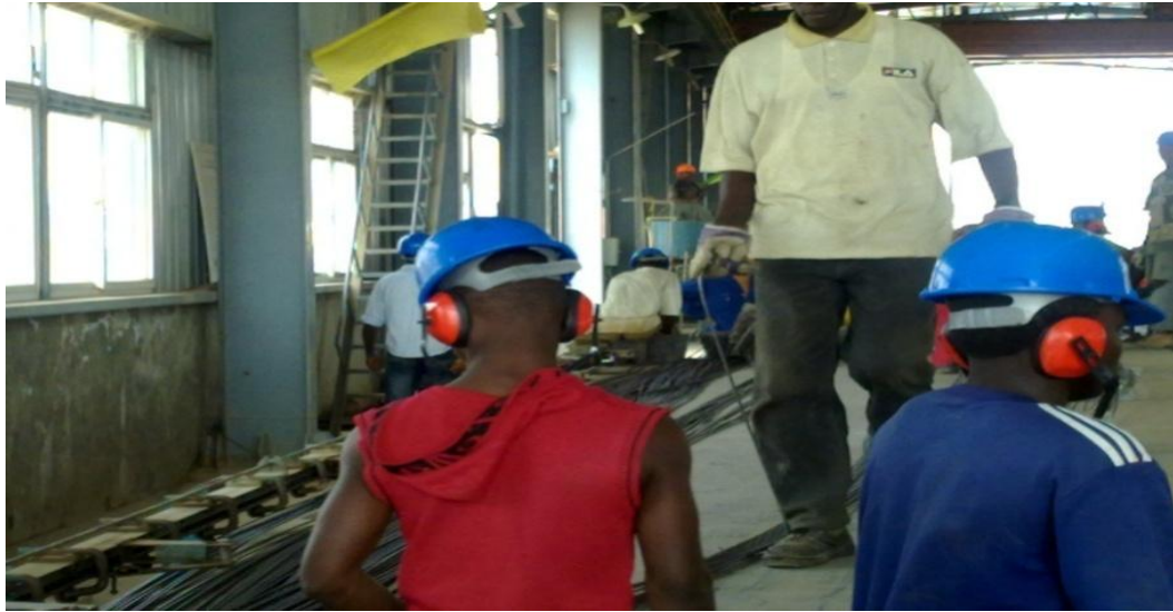
Picture 10: Ongoing work at Abuja Rail Transport station
