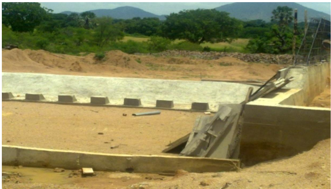
Picture 4: Ongoing bridge construction works at the Gombe Bypass
