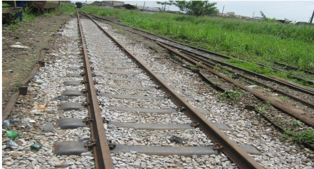
Picture 15: Newly laid track in Lagos Area (3.6 Guage): Lagos – Jebba Rail Line
