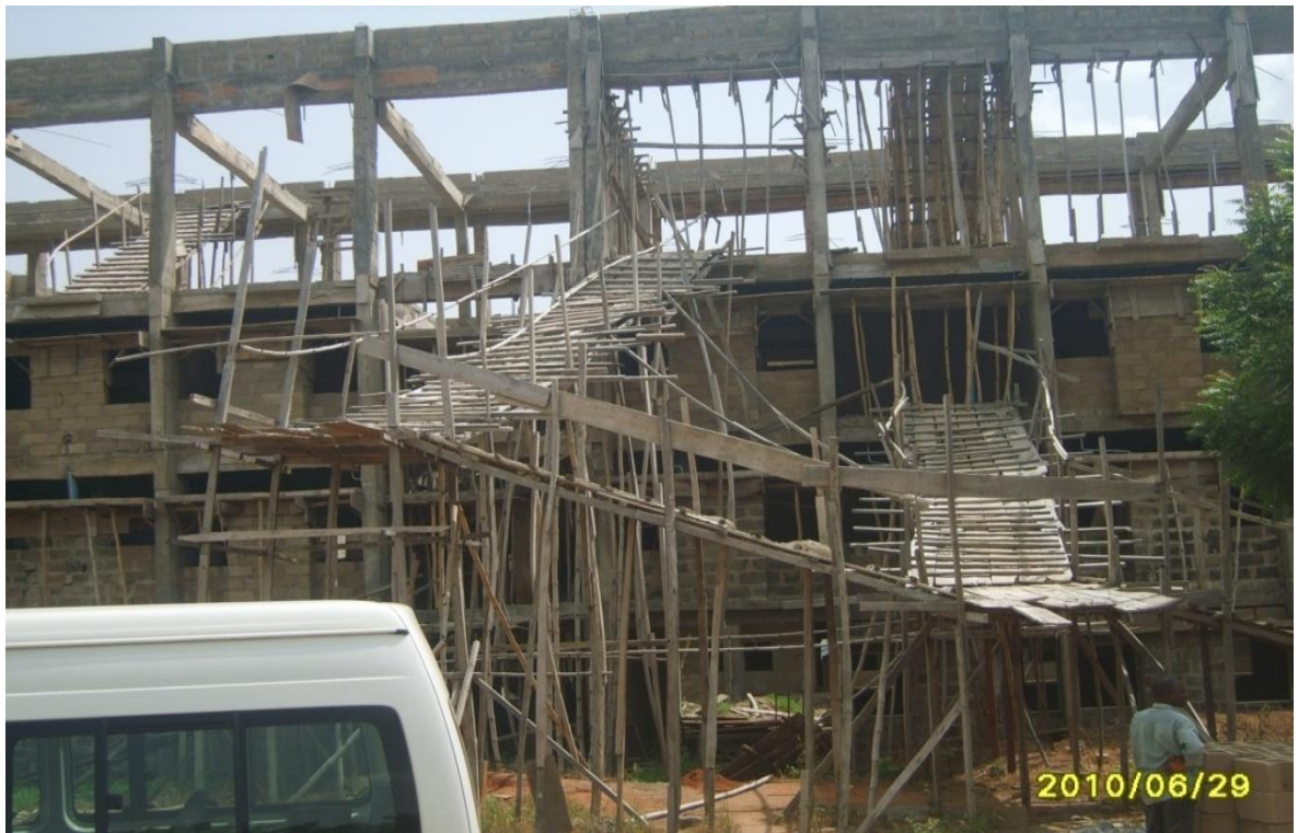
Picture 13: On-going Construction of COHS/BSS (ICT) at the University of Ilorin
