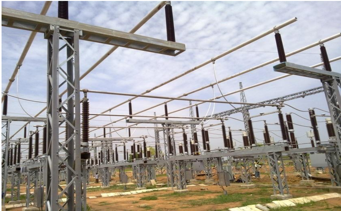
Picture 17: Ongoing work on the Damaturu sub-station
