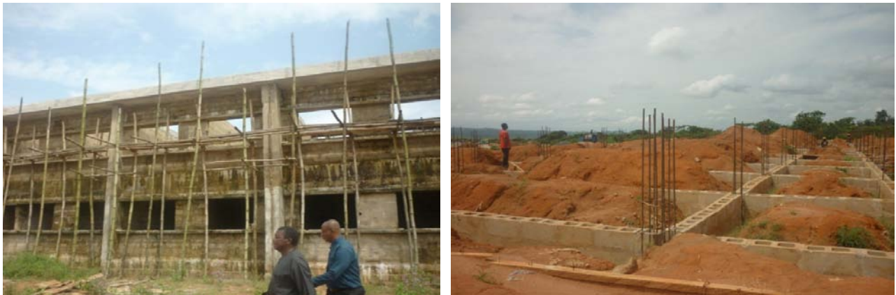
Picture 13: Construction of Specialty Clinic and Male Surgical Ward
