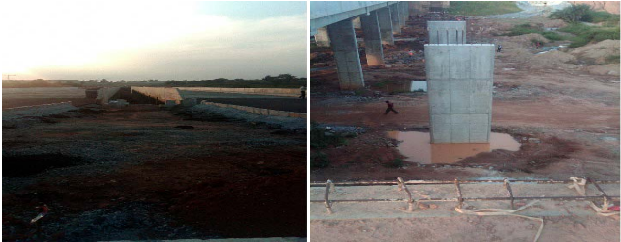
Picture 2: Ongoing Works in Idu Development District
