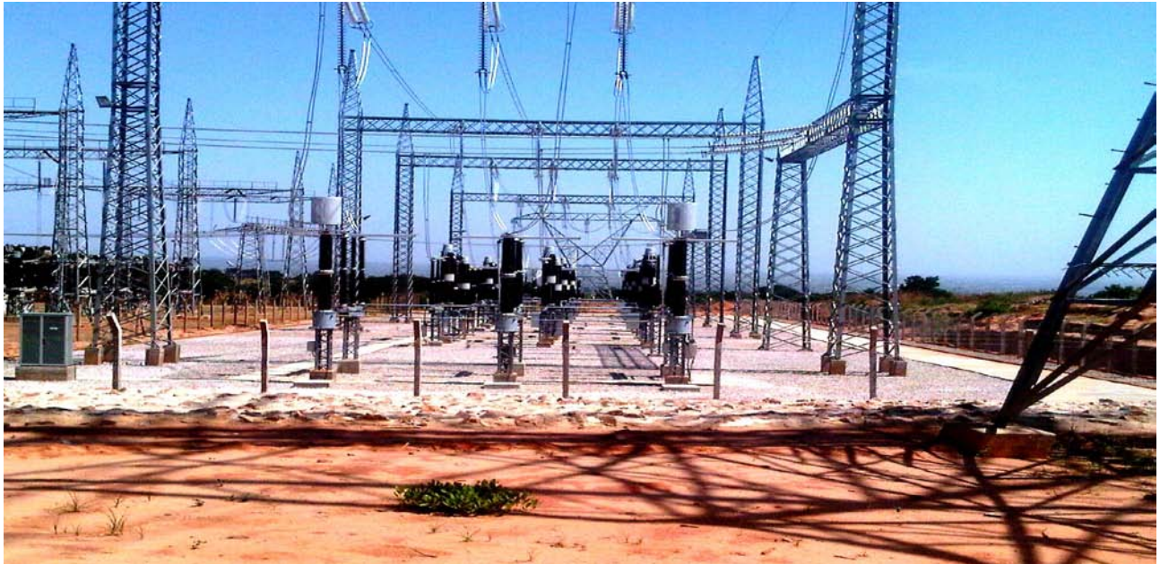
Picture 21: Ongoing Electricity work at Bay Extension at Gombe
