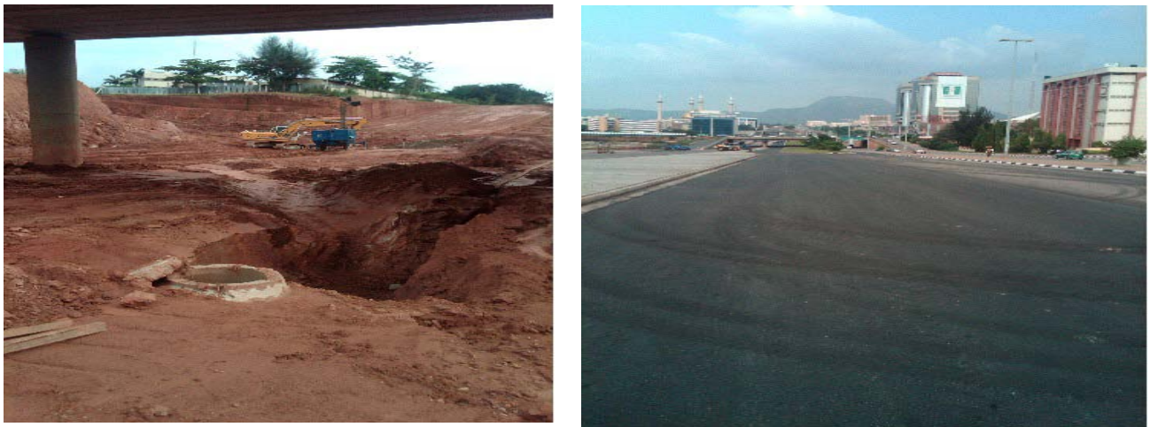
Picture 3: Flyover Bridge & Channelization Work at Mogadishu Cantonment
