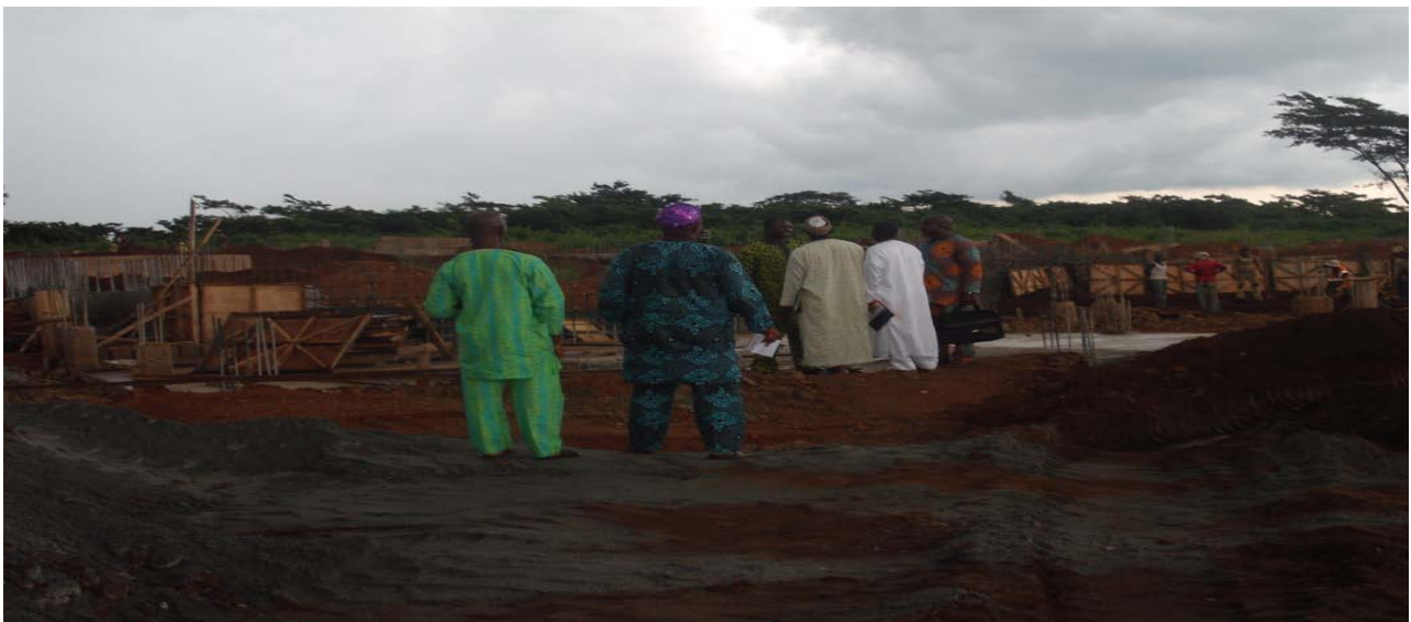
Picture 8: Construction of 2,500 Seater Auditorium at UNAAB
