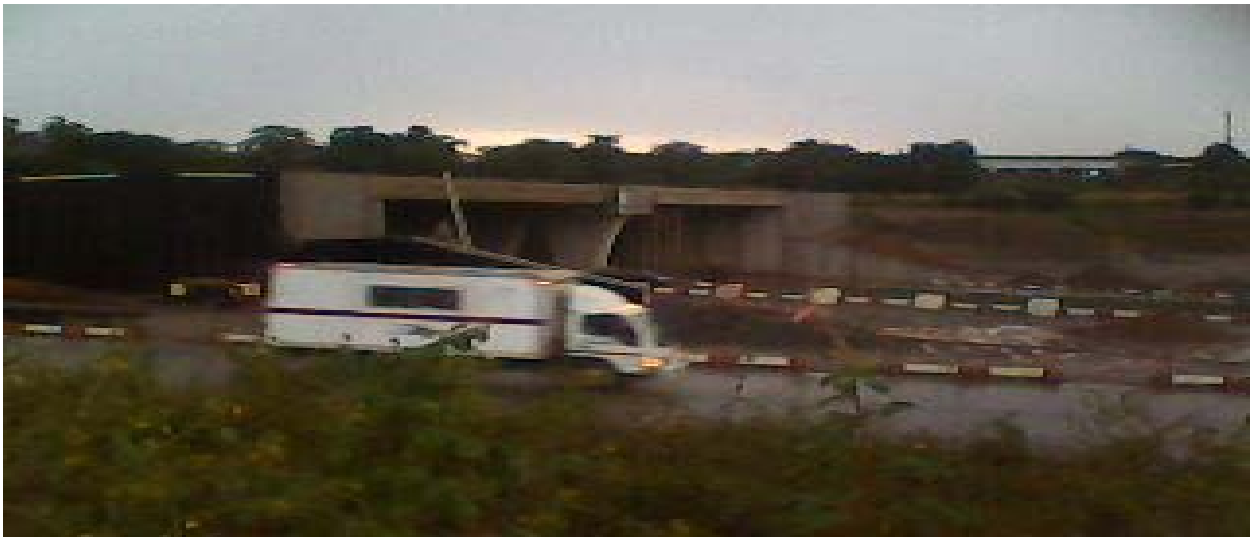
Picture 4: Flyover Bridge under construction along AYA-Keffi Dual carriageway
