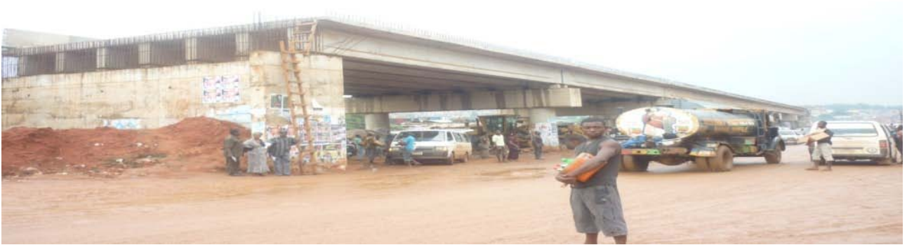
Picture 25: Onitsha – Enugu bypass through Obosi to join Onitsha – Owerri Road
