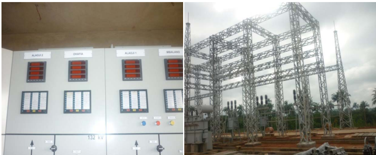
Picture 20: Completed Control Protection Panel Erection and Installation of 33KV Equipment.
