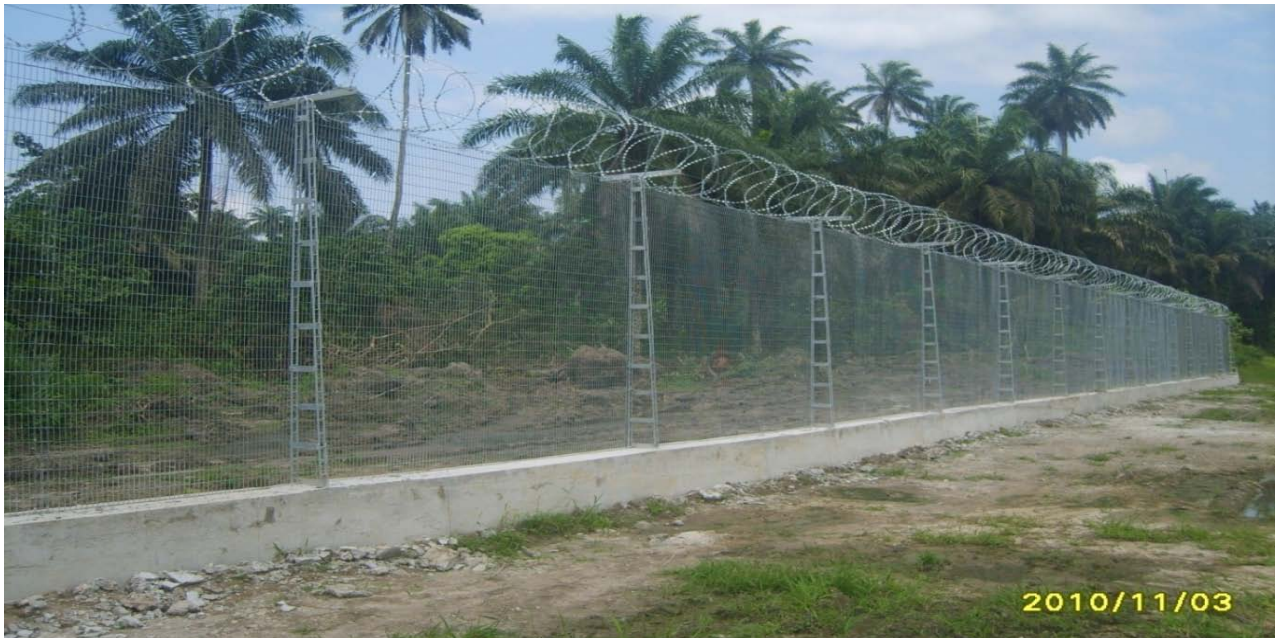
Picture 28: One of the Side-Views of Constructed Boundary Fence at Port-Harcourt International Airport
