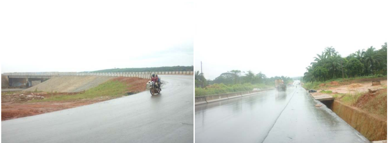
Picture 24 (a & b): Interchange at Obosi, & Ongoing works at Onitsha-Nkpor Road
