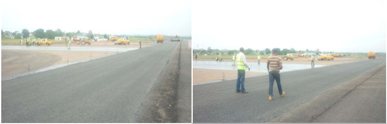
Picture 29: Ongoing Work at Enugu Airport
