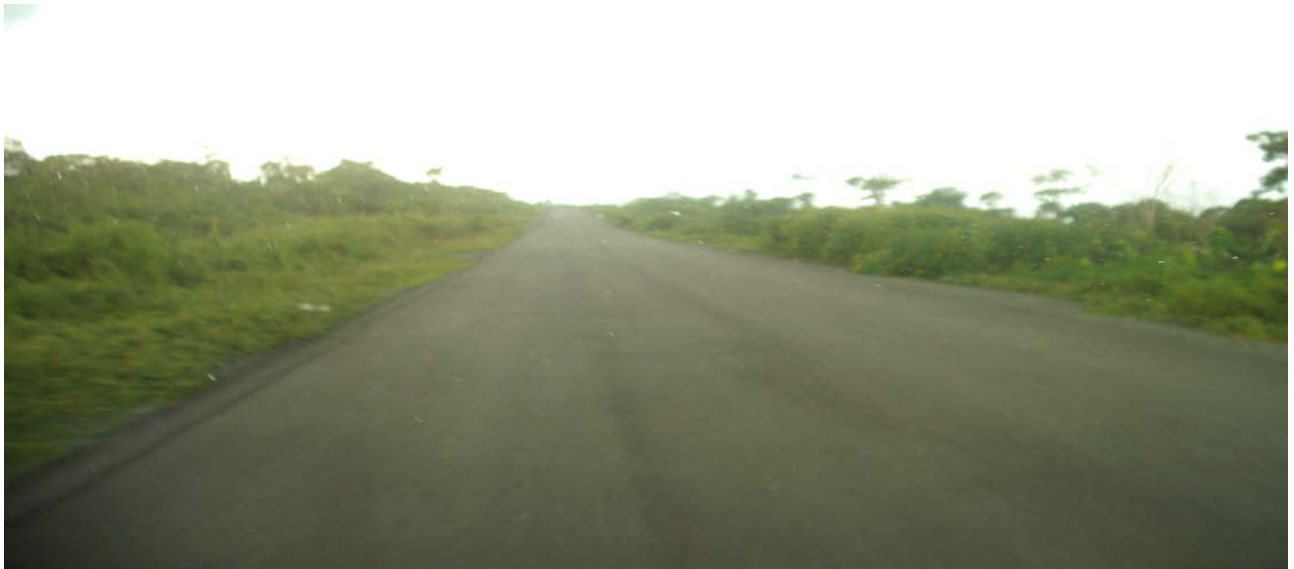
Picture 23: Construction of Ijebu-Igbo Sekono Road, Ogun State.
