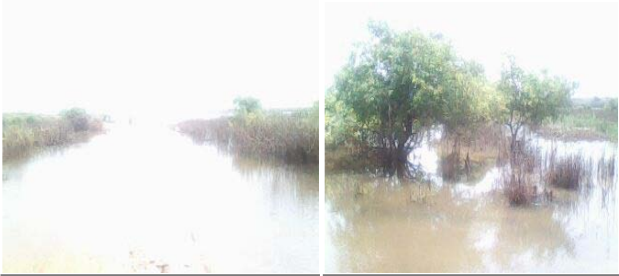
Picture 31: Flooding areas at Tada-Shonga Dam, Ilorin
