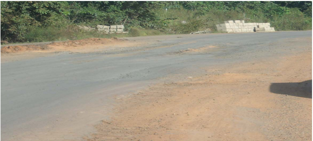
Picture 22: Rehabilition of Akungba-Ikare Road.
