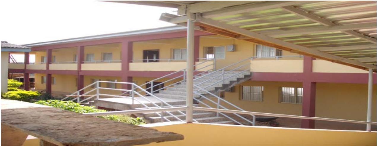
Picture 12: Completed Clinical Consulting Block
