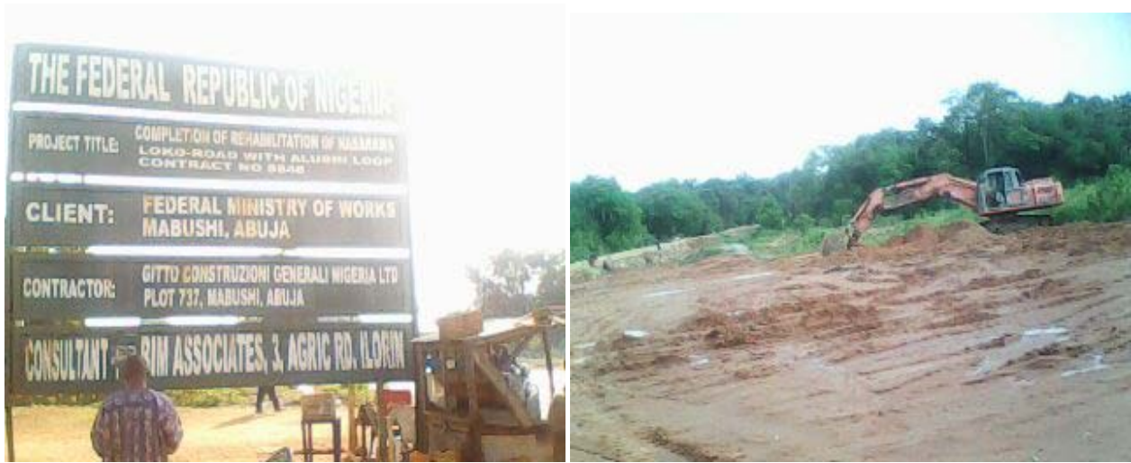
Picture 27 (a & b): Nasarawa-Loko Road under construction
