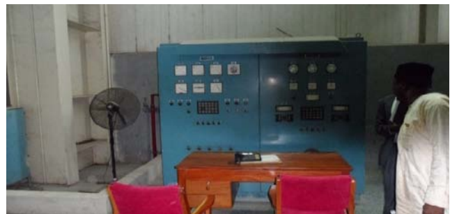
Picture 30: The rehabilitated Unit 1G7 and its Auxiliaries, Phase II
