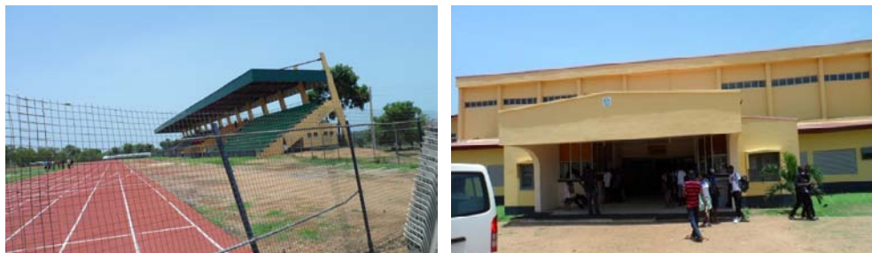
Picture 39: Completed Sports Complex at the University of Ilorin.
