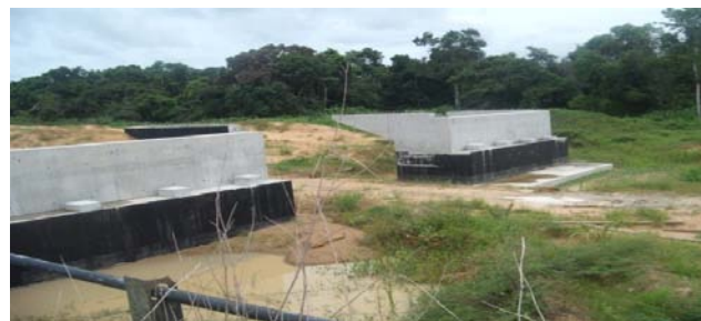
Picture 2: East-West road section 11 (PH –Kaiama) - Ongoing bridgework
