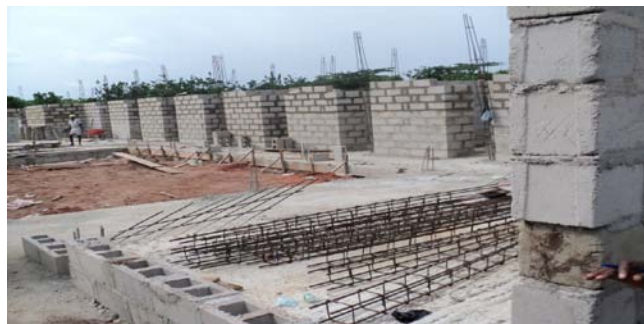
Picture 18: Construction of Students' Hostel in progress at the College
