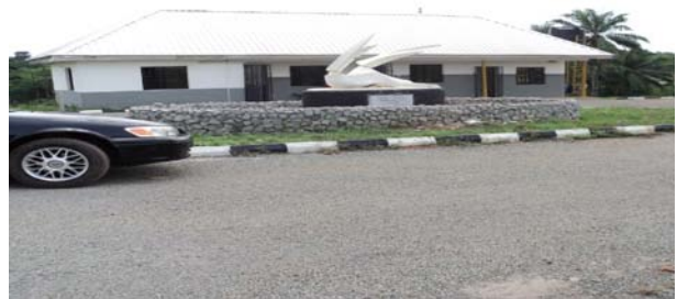
Picture 35: Completed water works office/access road at the Hospital
