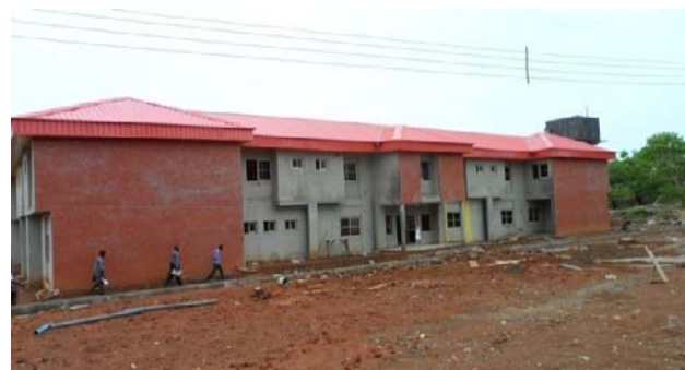
Picture 21: The Trainee Hostel Block/Conference Centre almost completed.
