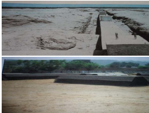
Picture 4: The Inland River Port, Baro under construction
