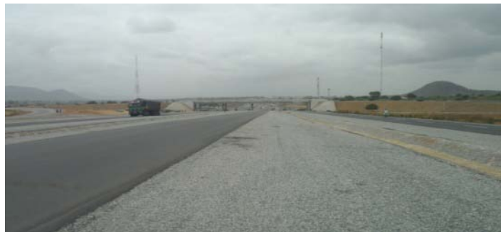
Picture 24: Section I Abuja-Abaji Road under construction
