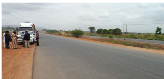
Picture 25: On-going construction of Section II, Abuja – Lokoja Road
