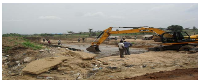
Picture 29: Completed Underpass and an on going work on the Project
