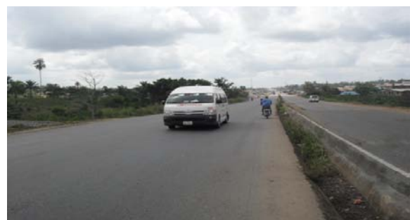
Picture 27: Completed Portion of the Shagamu – Ajebandele Ore Road, Section 1
