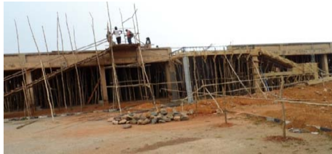
Picture 33: HIV Centre under construction at University of Jos Teaching hospital
