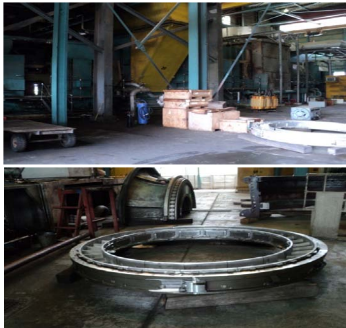
Picture 31: Rehabilitation of GT17 & spares for GT18 & GT 20, Ughelli Power Station.
