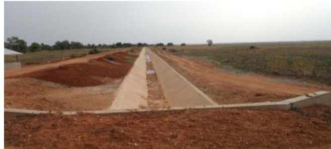
Picture 13: Wushishi Dam Irrigation component almost completed.
