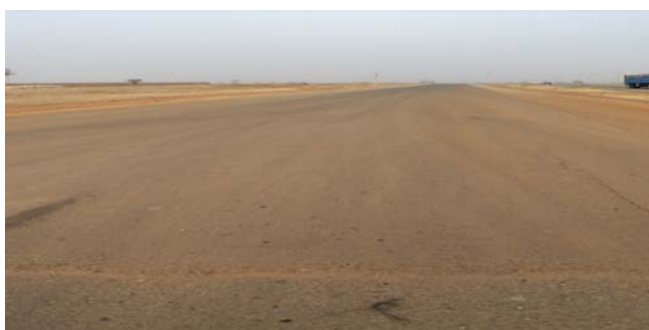
Picture 26: On-going Dualization of Kano-Maiduguri Road Section IV: Potiskum -Damaturu
