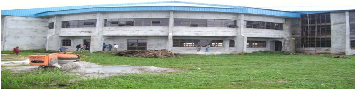
Picture 4.13: Ongoing Construction of 300 Seat Library /Resources Centre, Oron
