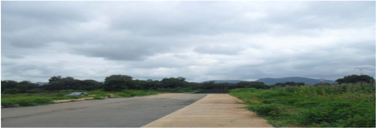
Picture 4.3(a): Completed asphalt overlay at Dutse Baupa- Bwari Road
