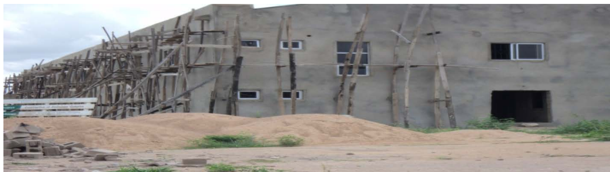
Picture 4.26: Ongoing-going Construction of Radiology Complex at FMC, Azare
