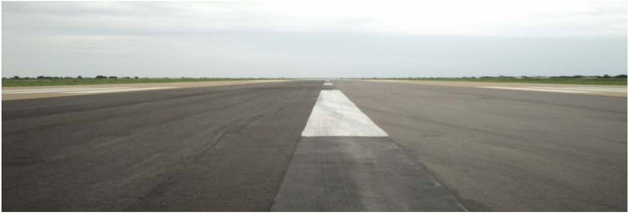
Picture 4.20: Completed 3 km runway at Maiduguri International Airport.
