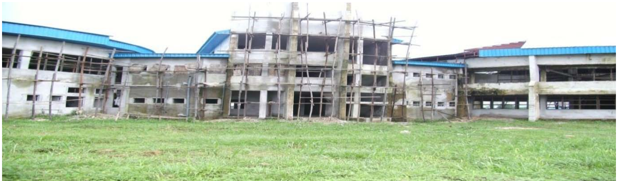
Picture 4.12: Construction of 1000 -Seat Auditorium at Maritime Academy, Oron
