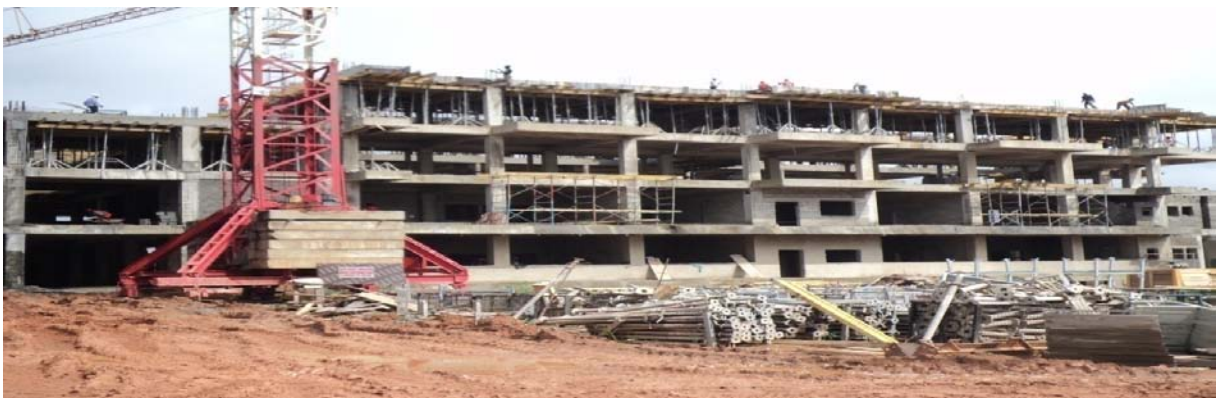
Picture 4.29: Ongoing-going construction works of PSC Corporate Headquarters
