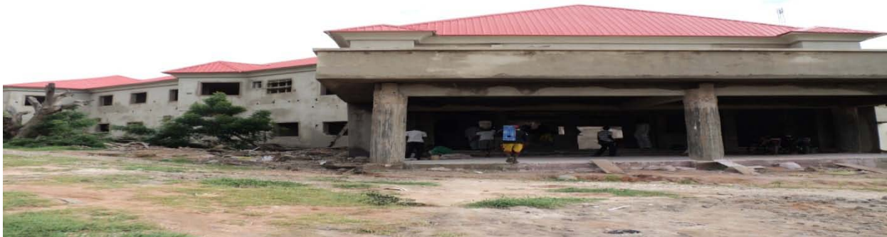
Picture 4.35: Construction of an Office Complex at FCE, Gombe
