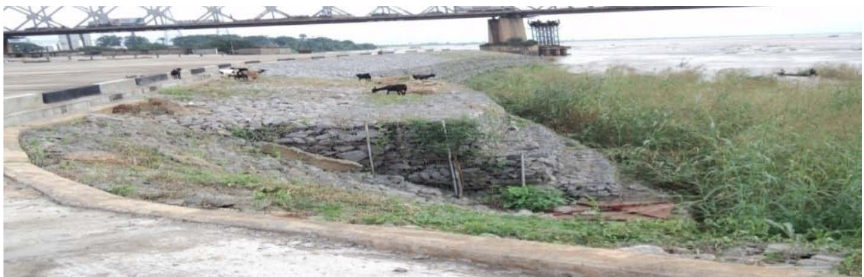
Picture 15(b): Completed shore line protection.
