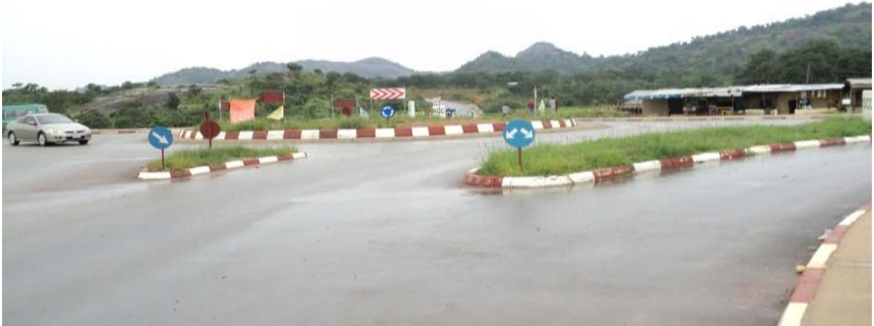
Picture 4.4: Newly constructed roundabout, a section of the re-construction of Lower Usuma Dam – Gurara Dam Road
