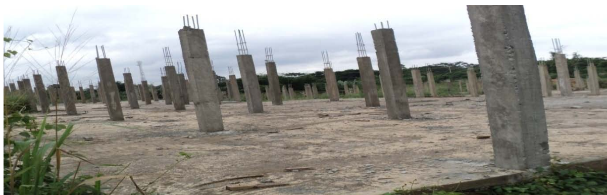
Picture 4.28: Ongoing Construction of Accident and Emergency Complex at FMC, Owo
