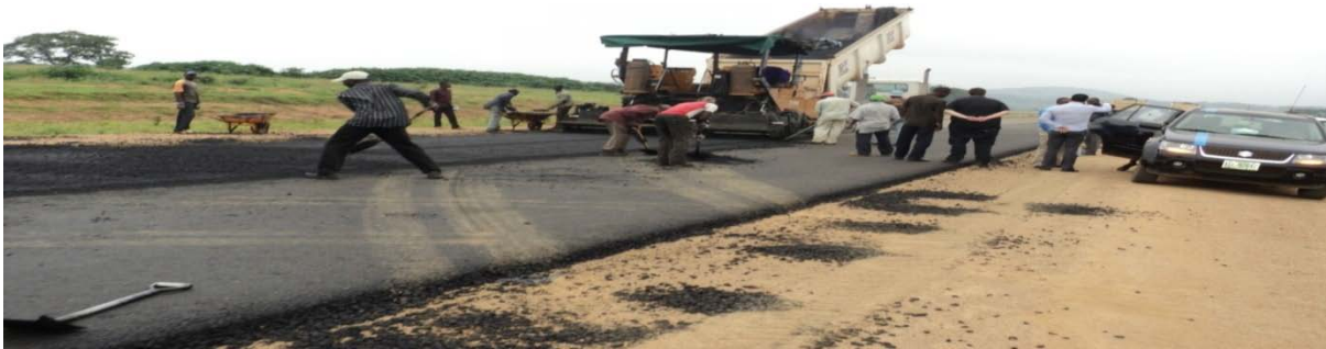
Picture 4.7: Ongoing construction work of the dualization of Ibadan – Ilorin Road (Route A2) Section II: Oyo – Ogbomosho Road
