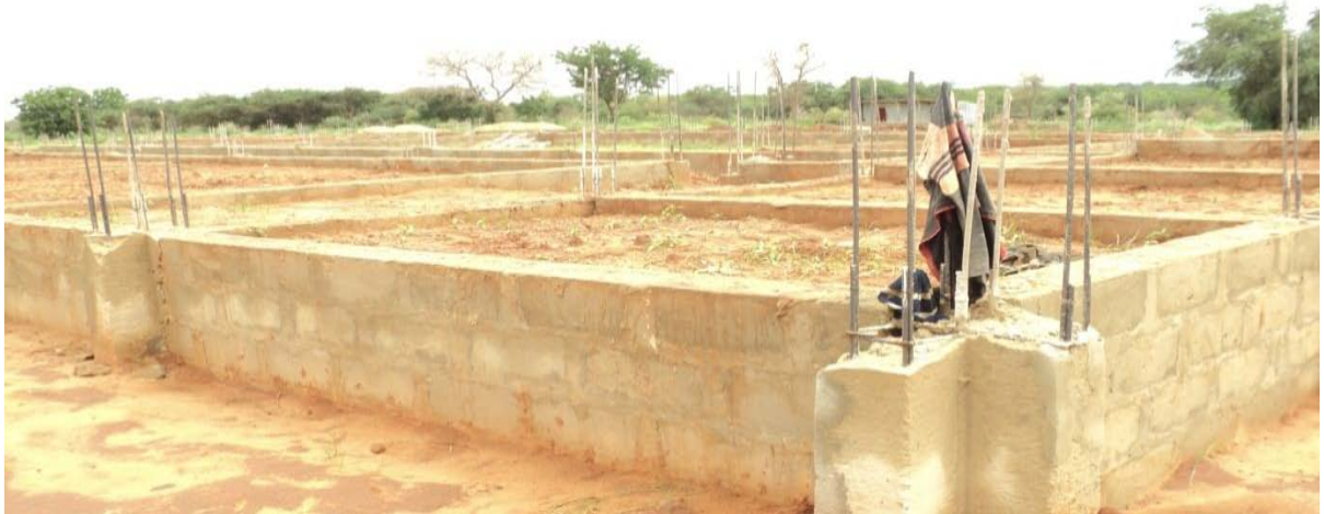
Picture 4.23: Ongoing-going construction of Multi-purpose Continental Lecture Hall at the site
