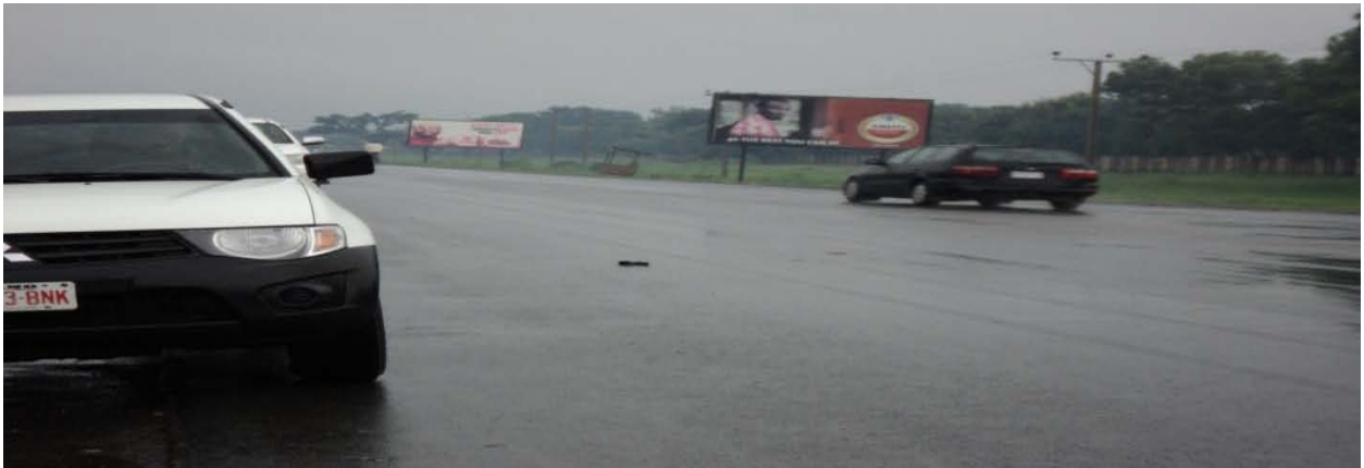
Picture 4.6: Completed wearing course at Bauchi-Dass-Tafawa Balewa Road
