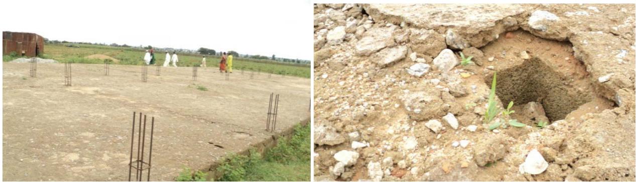
Picture 4.30(a): DPC work at the site of the Administrative Block
