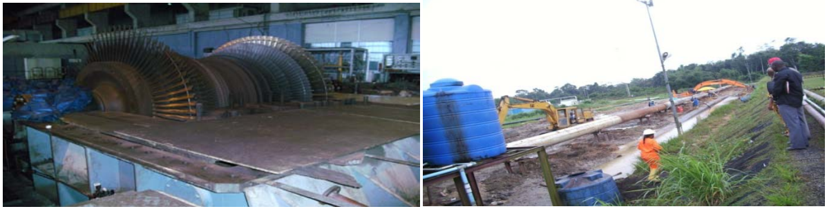
Picture 4.42: Ongoing Repairs to the Gas pipeline at Sapele Power Station
