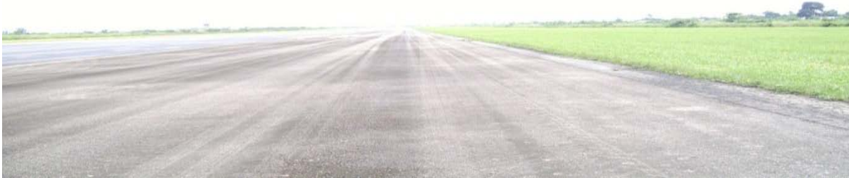
Picture 4.21: Runway extension/resurfacing work at Calabar, Airport
