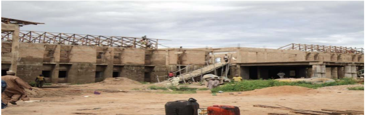
Picture 4.33: Construction of Male Hostel at FCE, Gombe
