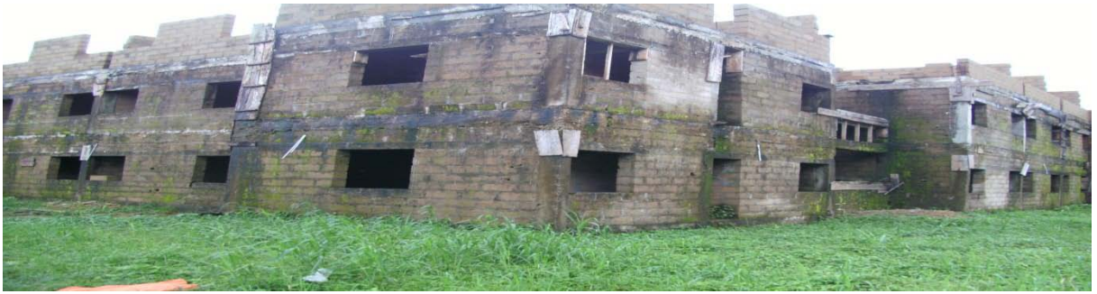
Picture 4.14: Ongoing Construction of 200 Capacity Male Cadet Hostel at Oron
