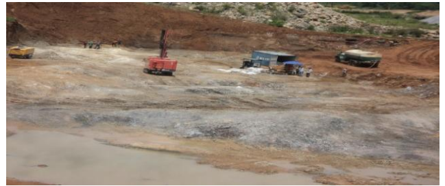
Picture 8: Assembling of pre-cast trash track of hydropower in-take & grouting of the foundation for the dam in progress at Kashimbilla Dam
