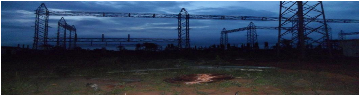
Picture 22: On-going work at Ohafia Sub-station, Abia state.
