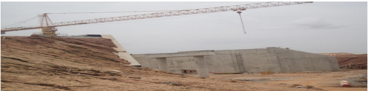
Picture 1: On-going Construction of Railway crossing bridges at (ONEX) Lot 1
