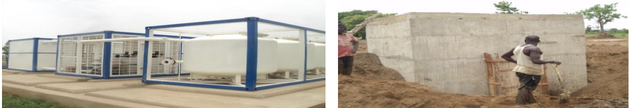
Picture 17: Water Treatment Plant and Reservoir almost completed at the site
