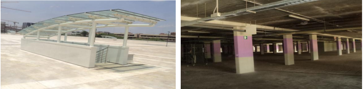
Picture 2: A portion of the completed National Square and Parking area at the project site
