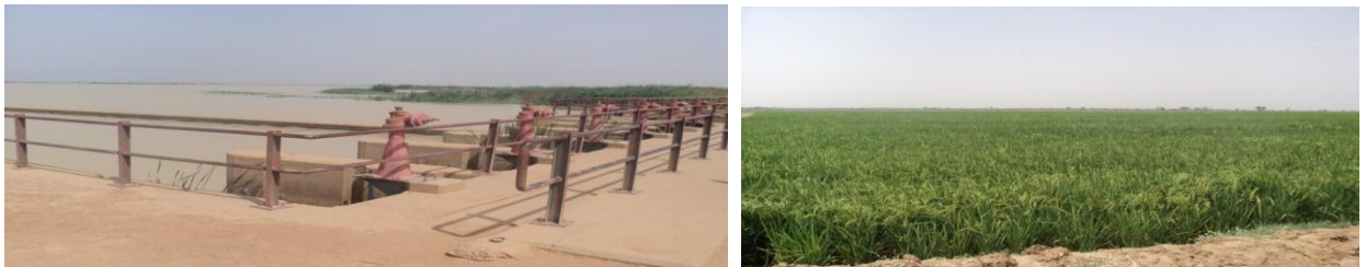
Picture 7: Completed distributor canal and Rice farm at Hadejia Valley Irrigation Scheme Project
