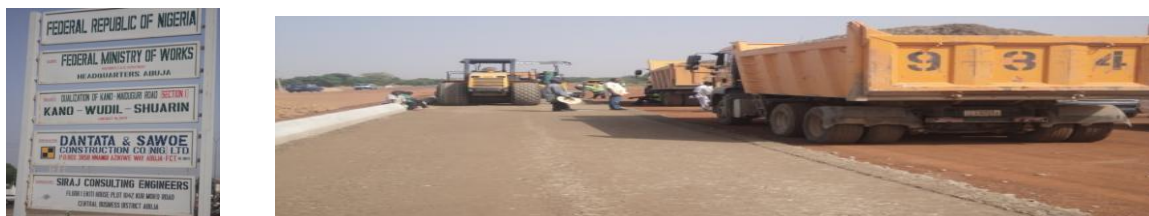
Picture 4: Ongoing construction work at Kano – Maiduguri Road (Kano – Wudil – Shuarin)
