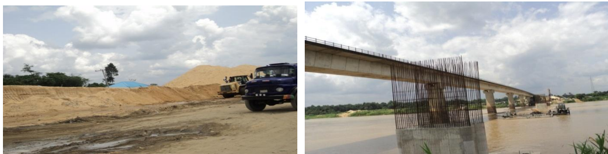
Picture 15: On-going earthworks and Abutment works at Kaiama bridge
