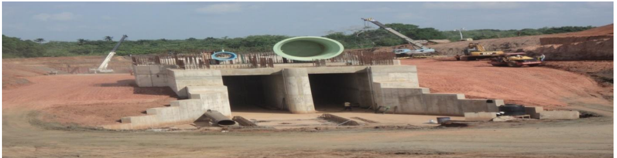
Picture 11: Installation of intake bell mouth at Otukpo Multi-purpose Dam.
