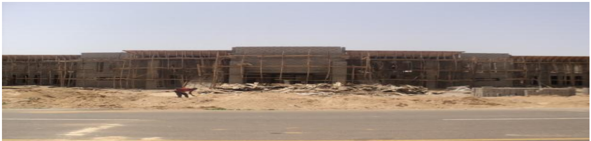
Picture 16: On-going construction of Biotechnology Research Centre, Bayero University Kano
