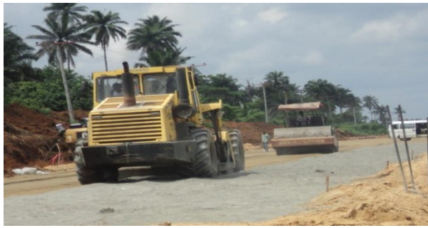
Pictures 14: Laying of stone base and Asphaltic Binder works in progress at Port-Harcourt– Ahoada,
