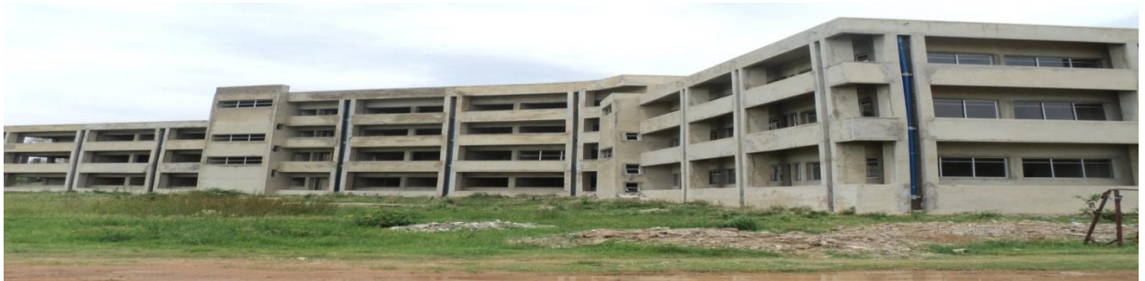
Picture 20: Ongoing Construction of Administrative Block/Senate Chamber University of Jos.
