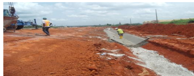
Picture 5: Flag off and on- going work of Trapezoidal shape drainage at section 1 of Lagos – Ibadan.
