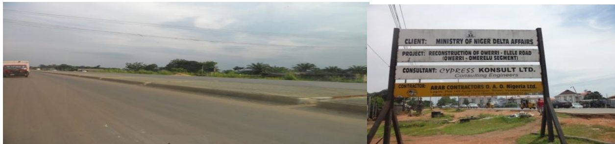
Picture 12: Completed portion of Elele-Owerri road, Imo state
