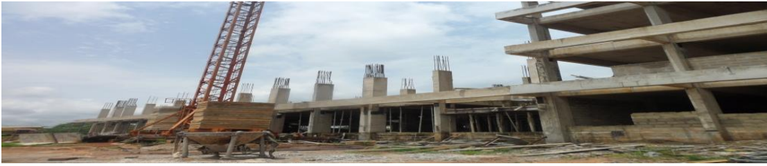
Picture 19: Ongoing Construction of Administrative building at UNN
