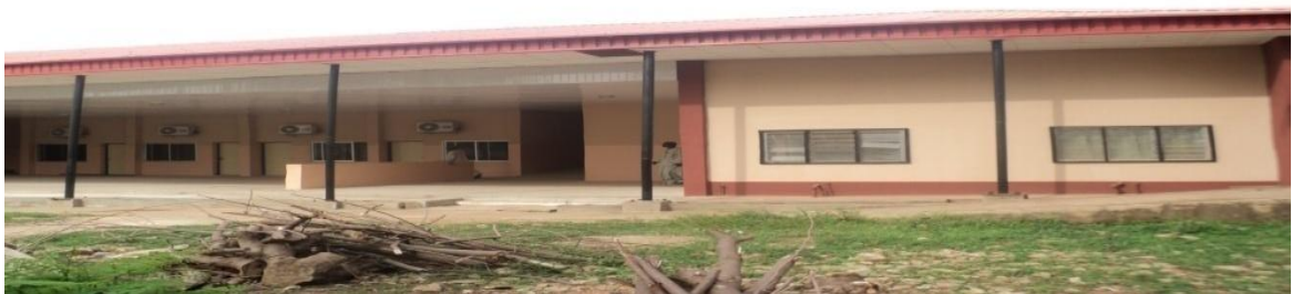
Picture 23: Rehabilitated GOPD at General Hospital Tudun Wada, ABUTH, Zaria.
