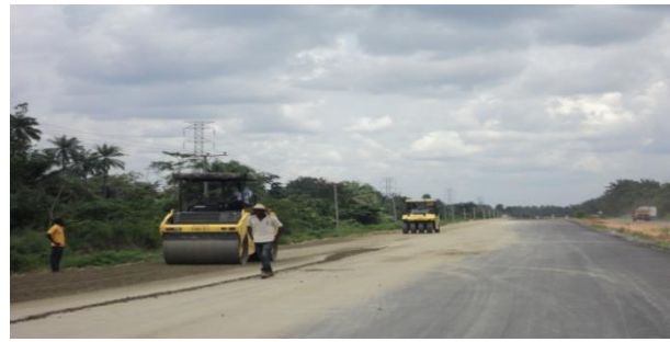
Pictures 14: Laying of stone base and Asphaltic Binder works in progress at Port-Harcourt– Ahoada,
