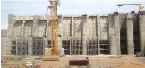
Picture 8: Assembling of pre-cast trash track of hydropower in-take & grouting of the foundation for the dam in progress at Kashimbilla Dam
