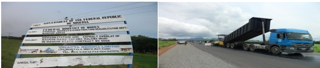
Picture 5: Ongoing work on Bauchi-Dass-Tafawa Balewa road
