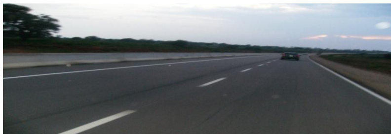
Picture 4: A completed portion of the dual carriageway (Kakau – Kachia)
