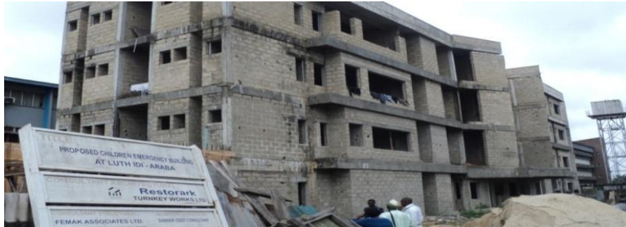
Picture 17: Ongoing Construction Work for Children Emergency Centre at LUTH.
