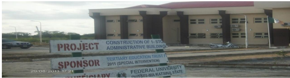
Picture 22: On-going Landscaping & drainage works around the Senate building complex
