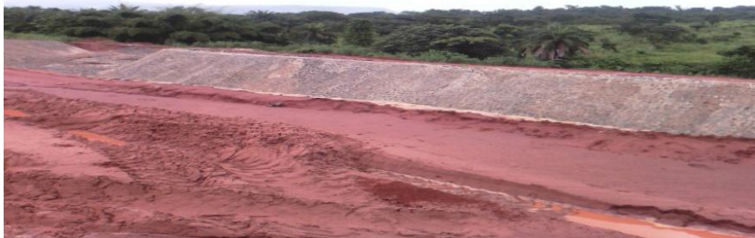
Picture 29: Stone pitching of spillway channel at Adada Dam
