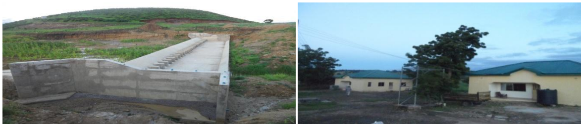
Picture 28: Completed spillway and permanent office/residential accommodation at Cham
