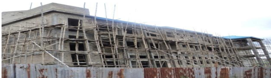
Picture 20: Admin building/Training Centre at roofing level
