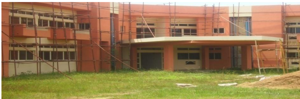
Picture 8: Participants' hostel complex almost completed at NITT, Zaria.
