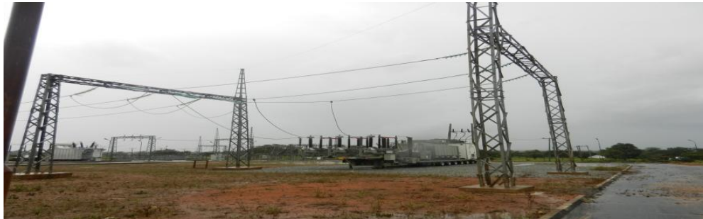
Picture 33: On-going construction of Akwanga – Lafia 132KV double circuit transmission line
