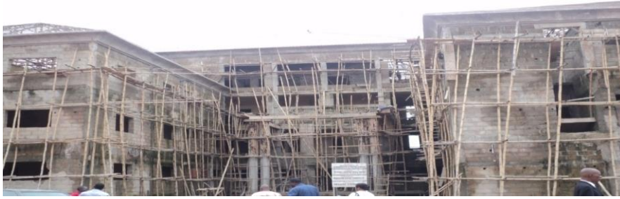
Picture 19: Construction of Administrative Building at NOFIC Abakaliki.
