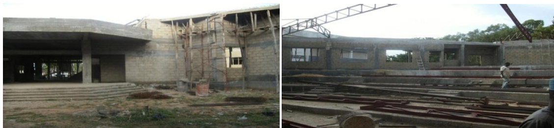
Picture 25: On-going construction of conference hall at IAR, Zaria
