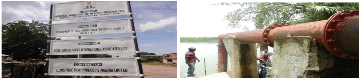
Picture 26: Part of the Completed Section of Tada - Shonga Irrigation Project
