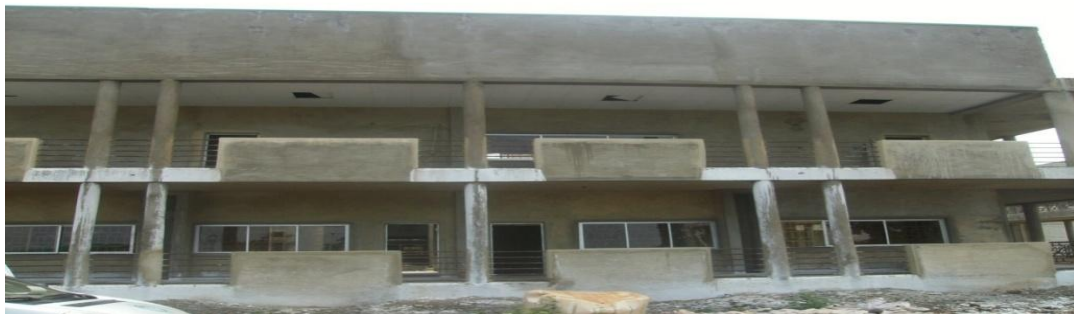
Picture 9: On-going Construction of Transport Technology Centre (TTC), Phase II
