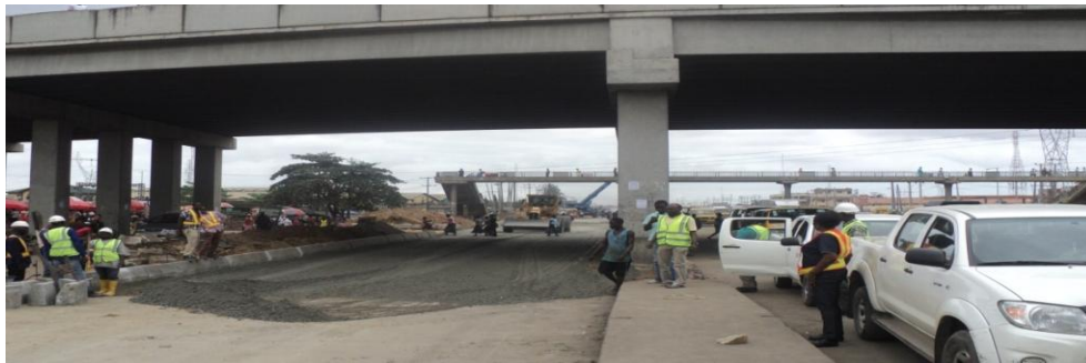
Picture 1: On-going Construction work at Apapa – Oshodi Expressway Section 2
