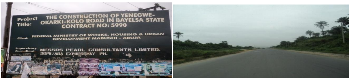
Picture 6: Construction of Yenegwe-Okaki-Okolo road in Bayelsa
