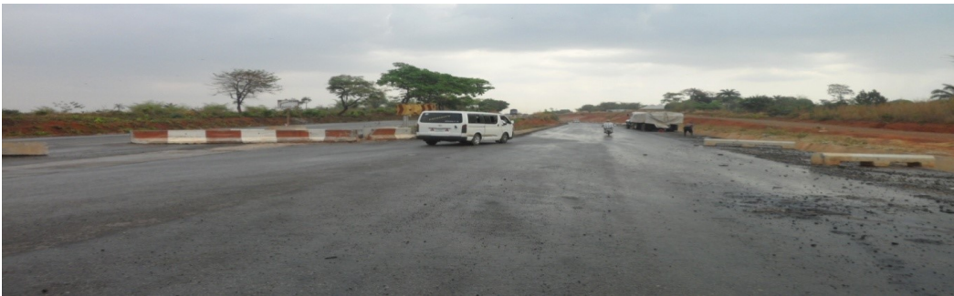
Picture 12: On-going Binder Course at Auchi-Ehor Junction, Section III
