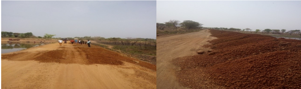
Picture 26: Construction Works in Progress at the Berugbum Dam Project
