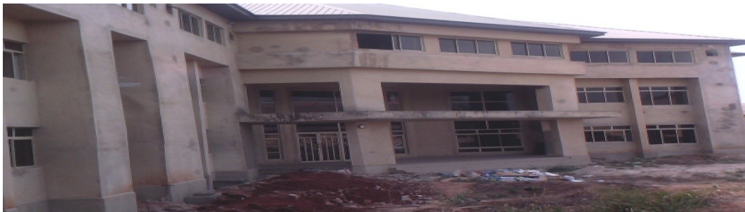
Picture 36: Ongoing Construction of Consulting Complex at FMC Umuahia
