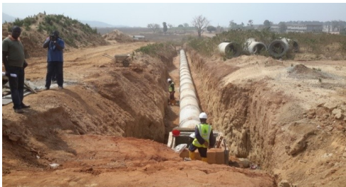
Picture 18: Laying of Storm Water Concrete Pipes & Stone Base at Kyami District, Abuja
