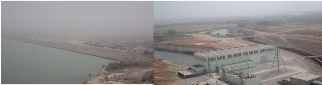
Picture 22: Completed Dam and Switchyard Substation Hydropower at Gurara Dam
