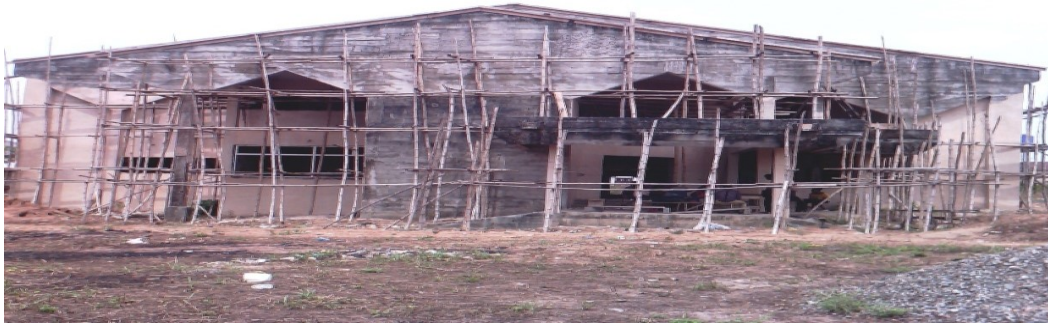
Picture 40: Ongoing Construction of School of Health Technology at FUT, Owerri
