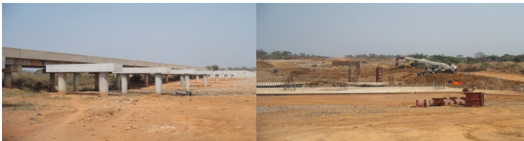
Picture 16: Construction of Piers in Progress at Usuma Dam Gurara Road
