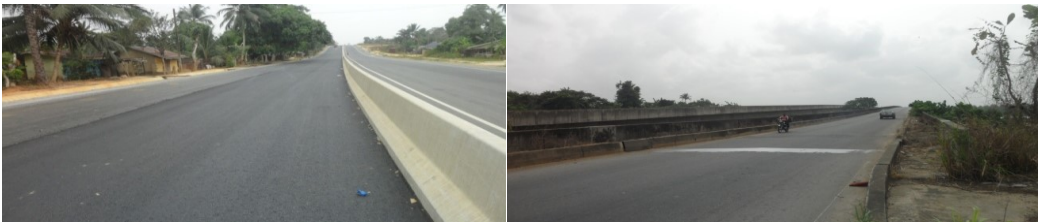
Picture 9: Ongoing Dualization of East West Road Section III (Port Harcourt-Eket)
