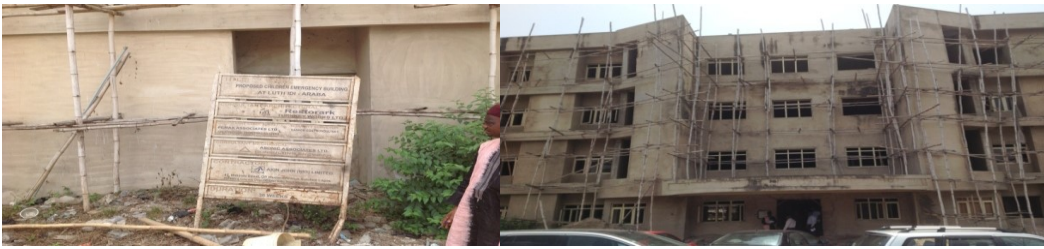
Picture 34: Ongoing Construction of Children Emergency Centre at LUTH, Lagos
