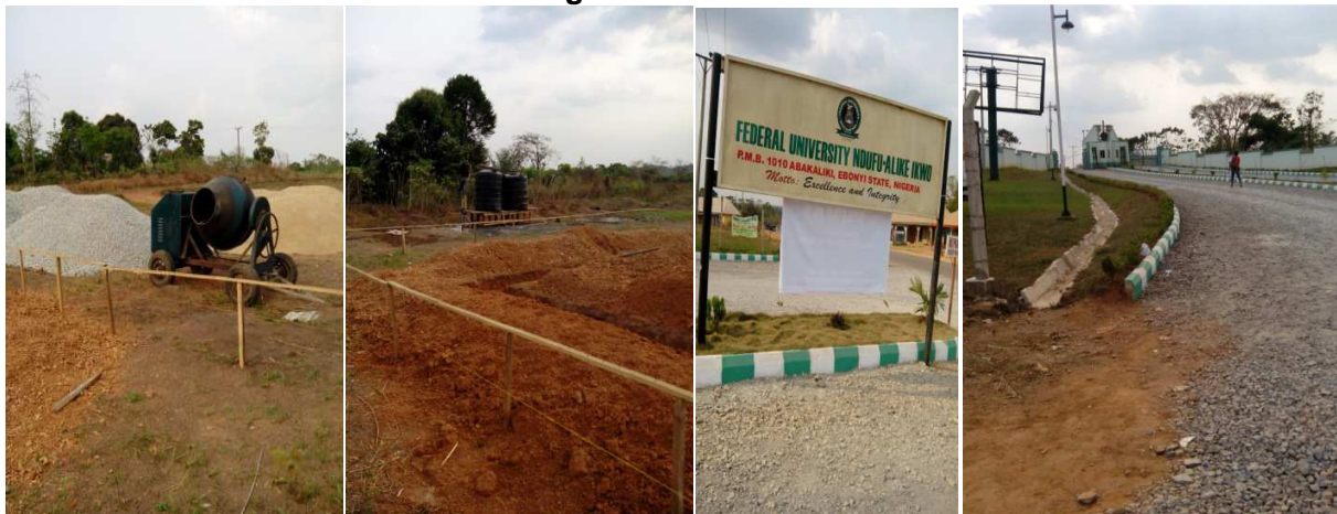
Construction of gate at Permanent Site
