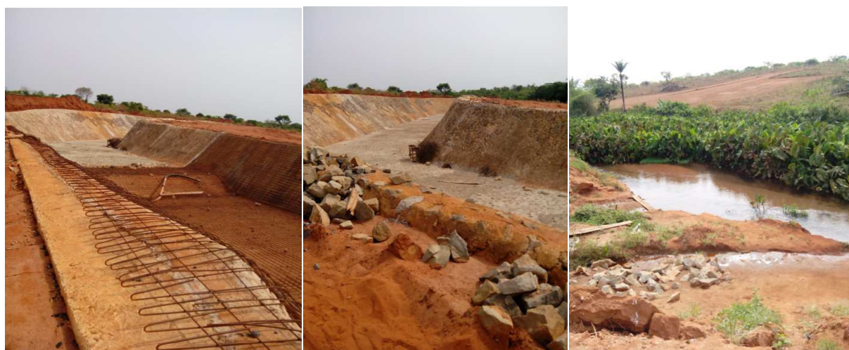
Meshing of the Spill Way Channel.
