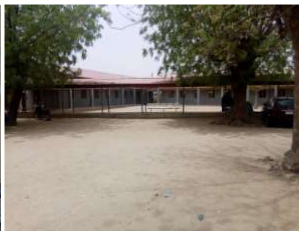
Picture 59: Front View of the PHCC
