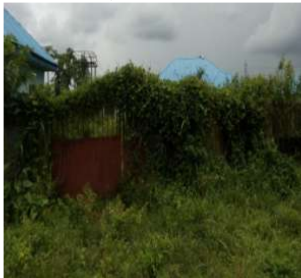
Picture 15: Completed but Abandoned Site
