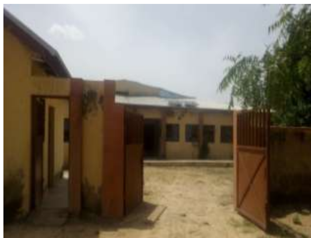
Picture 27: Front View of the PHCC
