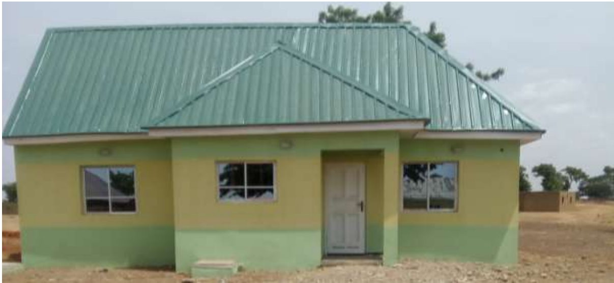
Picture 72: Primary Health Care Centre Kasuwa Magani
