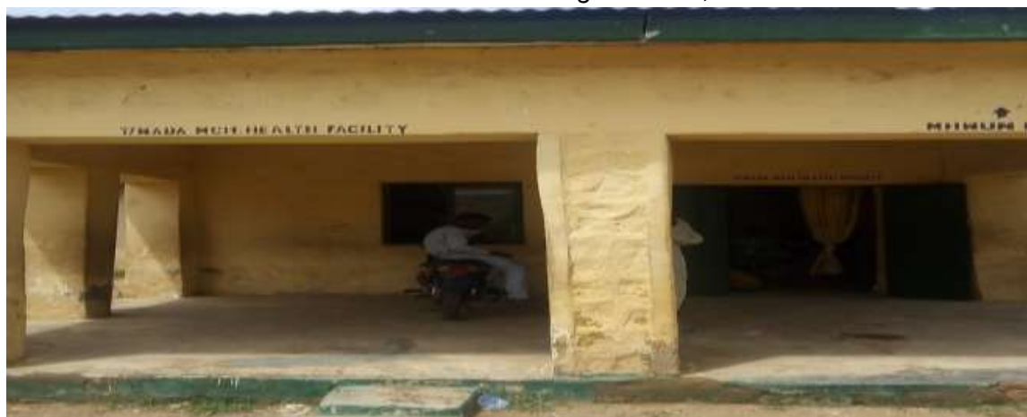
Picture 42: The Old Building of PHCC, Tudun Wada
