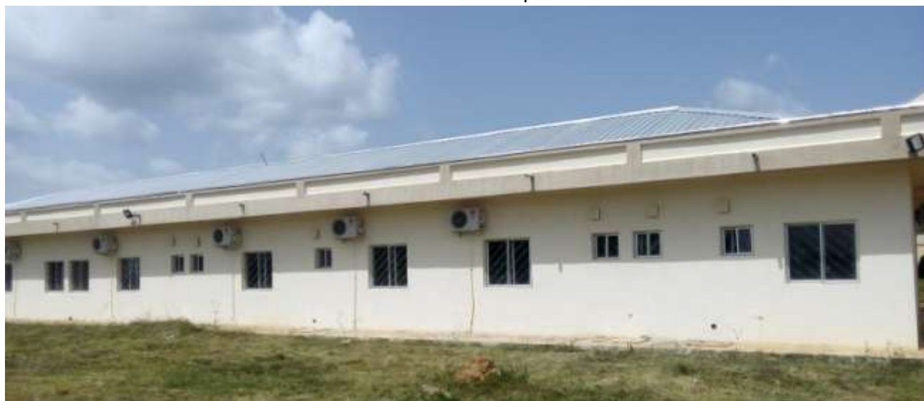
Picture 21: Back View of the Completed IVF Centre
