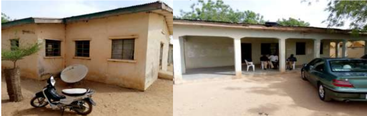
Picture 67: Facilities in the Old Building
