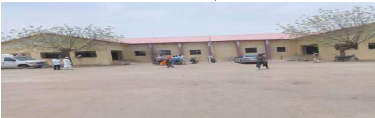
Picture 70: The Old Building, CHC Mashi
