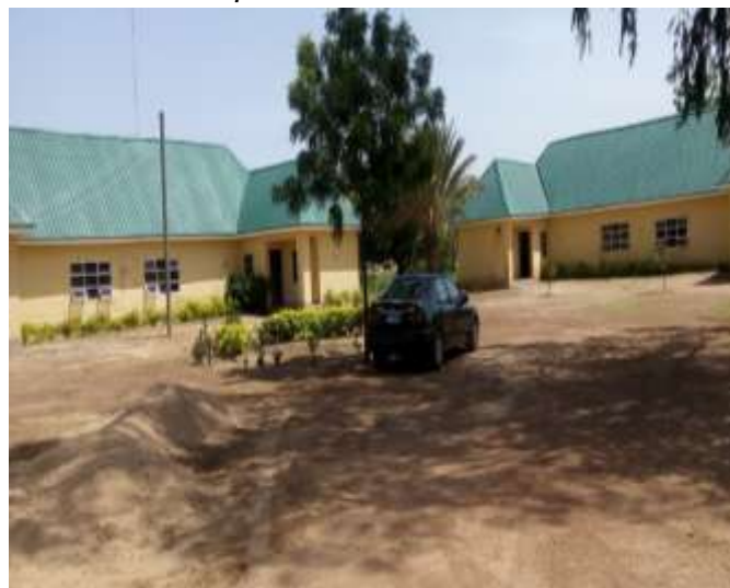
Picture 34: Completed Administrative Block
